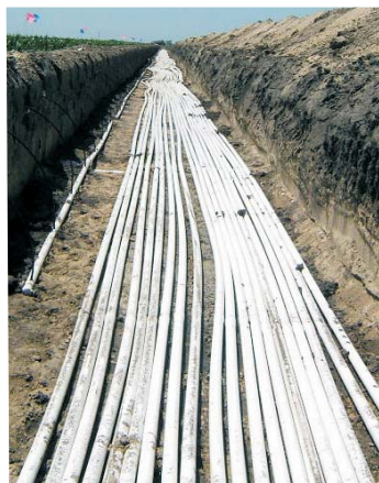
About 5 miles of 3-inch pvc pipe were installed to deliver variable rates of water to twenty treatments with three replications each.
