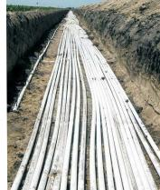
About 5 miles of 3-inch pvc pipe were installed to deliver variable rates of water to twenty treatments with three replications each.
