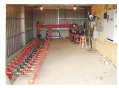
The SDI control unit includes: irrigation controller, variable speed controller, water and fertilizer flowmeters, chemical injection pump, along with numerous filters and valves.
