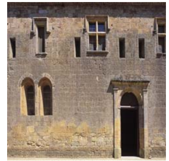
A4. Main door and adjacent windows
