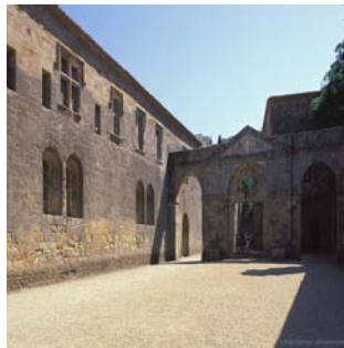
A2. Looking towards the back of the Court
