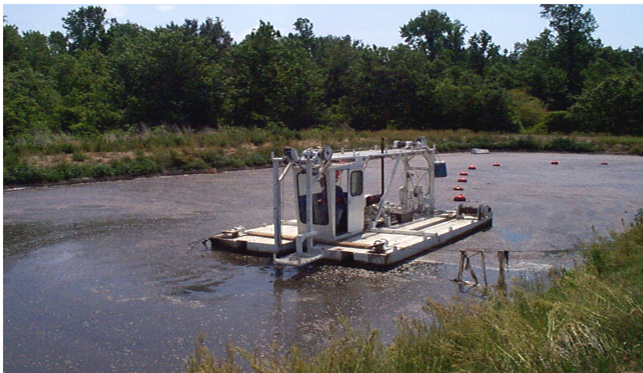
Figure 1. Pumping dredge operating in a lagoon in North Carolina.
