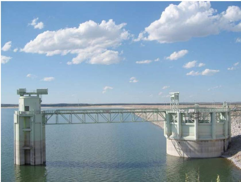
Photograph 2. Lake McConaughy in western Nebraska, a primary irrigation and recreational water source, has experienced record lows during recent drought. Note that the reservoir level is typically at the top of the water line shown on these structures. (Melissa Melvin, NDMC, 2006)
