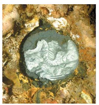
Figure 5. Surface of Arizona's hull after removal of a 76-mm (3-inch) diameter concretion disk and surface preparation. Note the unevenness of the surface, even after significant surface preparation. (Brett Seymour/NPS)
