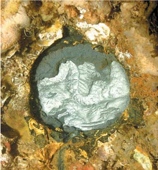
Figure 5. Surface of Arizona 's hull after removal of a 76-mm (3-inch) diameter concrete disk and surface preparation. Note the unevenness of the surface, even after significant surface preparation. (Brett Seymour/NPS)
