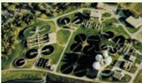
City of Lincoln “digesters” (above) process sewage into a suitable organic fertilizer for crops. Extension Technologist Dave Smith (right) takes soil samples to determine the amount of biosolids to apply per field. After transport to the fields (right center), the biosolids are applied to the fields (far right).
