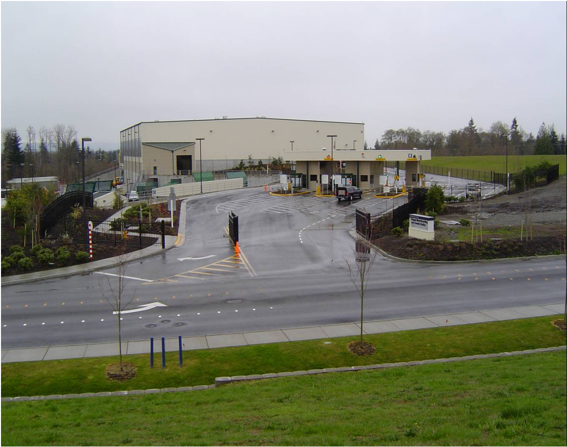
Figure 2. Photograph of the newly constructed and operational Airport Road Transfer Station at Paine Field, Washington.
