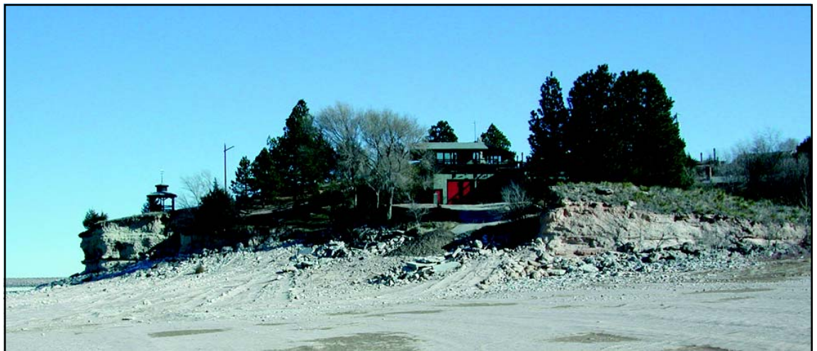
A fifth year of drought pulled Lake McConaughy down to 36 percent of capacity by the end of May and levels are continuing to decline. By the end of May, the lake was about 12 miles long and about 80 feet deep near Kingsley Dam. Many houses that formerly lined the lake's shoreline now appear as islands surrounded by sand (UNL School of Natural Resources photo).
