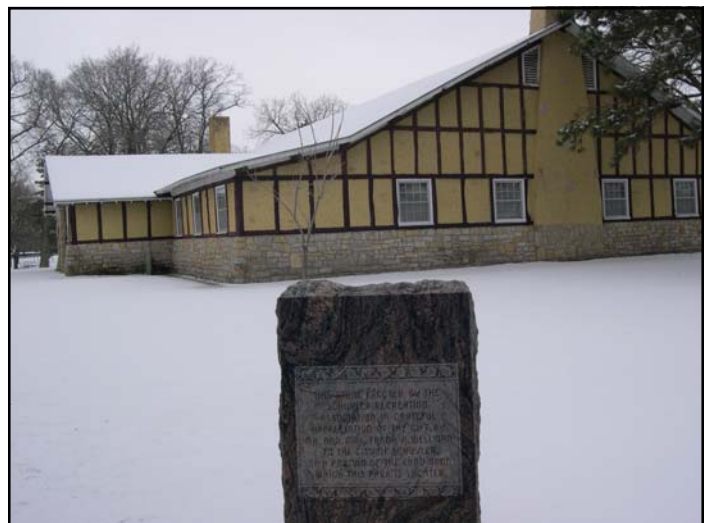
Schuyler's Oak Ballroom will be the site of a summer water and natural resources tour discussion of immigration and changing demographics that are affecting many communities in the Platte River Basin. The Work Project Administration built the ballroom in 1936 (photo: Rodney Verhoeff).
