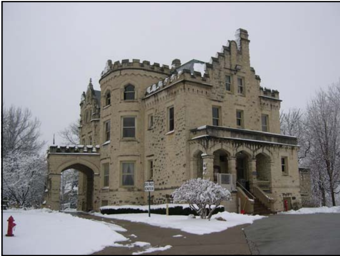
Omaha's Joslyn Castle, built just after the turn of the 20th Century, will be the backdrop for a summer water and natural resources tour presentation on promoting sustainable development by Cecil Steward of the Joslyn Castle Institute for Sustainable Communities (photo: Steve Ress).
