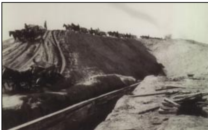
Muscle and determination helped build U.S. Bureau of Reclamation irrigation projects. Here, men and horses haul backfill material for sluicing into a cut-off trench at Minatare Dam in October, 1913. Additional copies of the October, 2002 Water Current giving the history of Bureau projects in Nebraska and eastern Wyoming are available free from the UNL Water Center (USBR photo).
