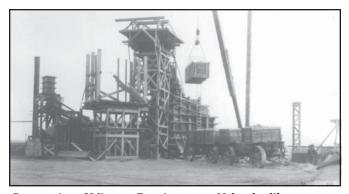
Construction of Minatare Dam in western Nebraska, like many early Reclamation projects, included having to elevate skips containing gravel into a hopper that screened the gravel. This photo
