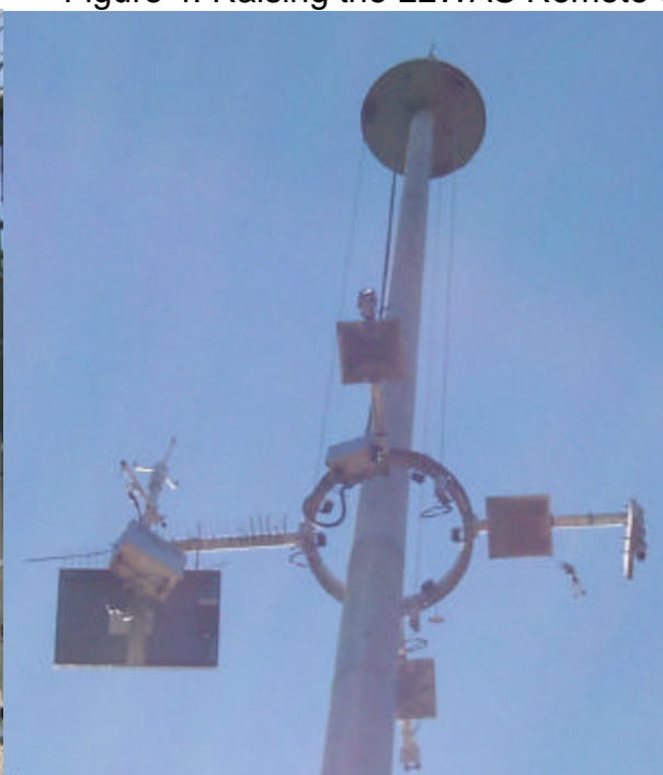
Figure 4. Raising the LLWAS Remote Station
