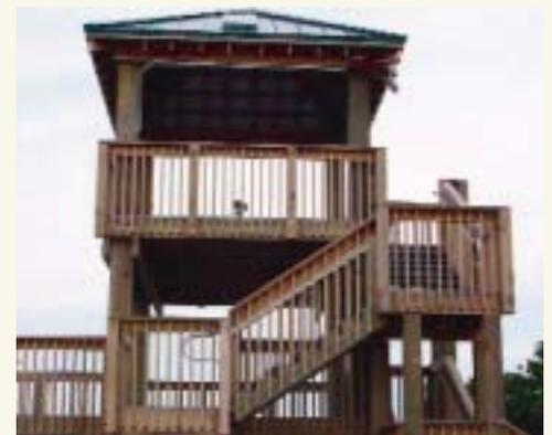
*J.N. “Ding” Darling NWR, FL, used fee monies to build an observation tower, redesigned to help comply with the Americans with Disabilities Act. The main level platform was expanded and an ADA-compliant ramp was installed. The refuge also completed rehabilitation on the Indigo Trail, installing a boardwalk with recycled plastic lumber and two rest benches. (USFWS)*
