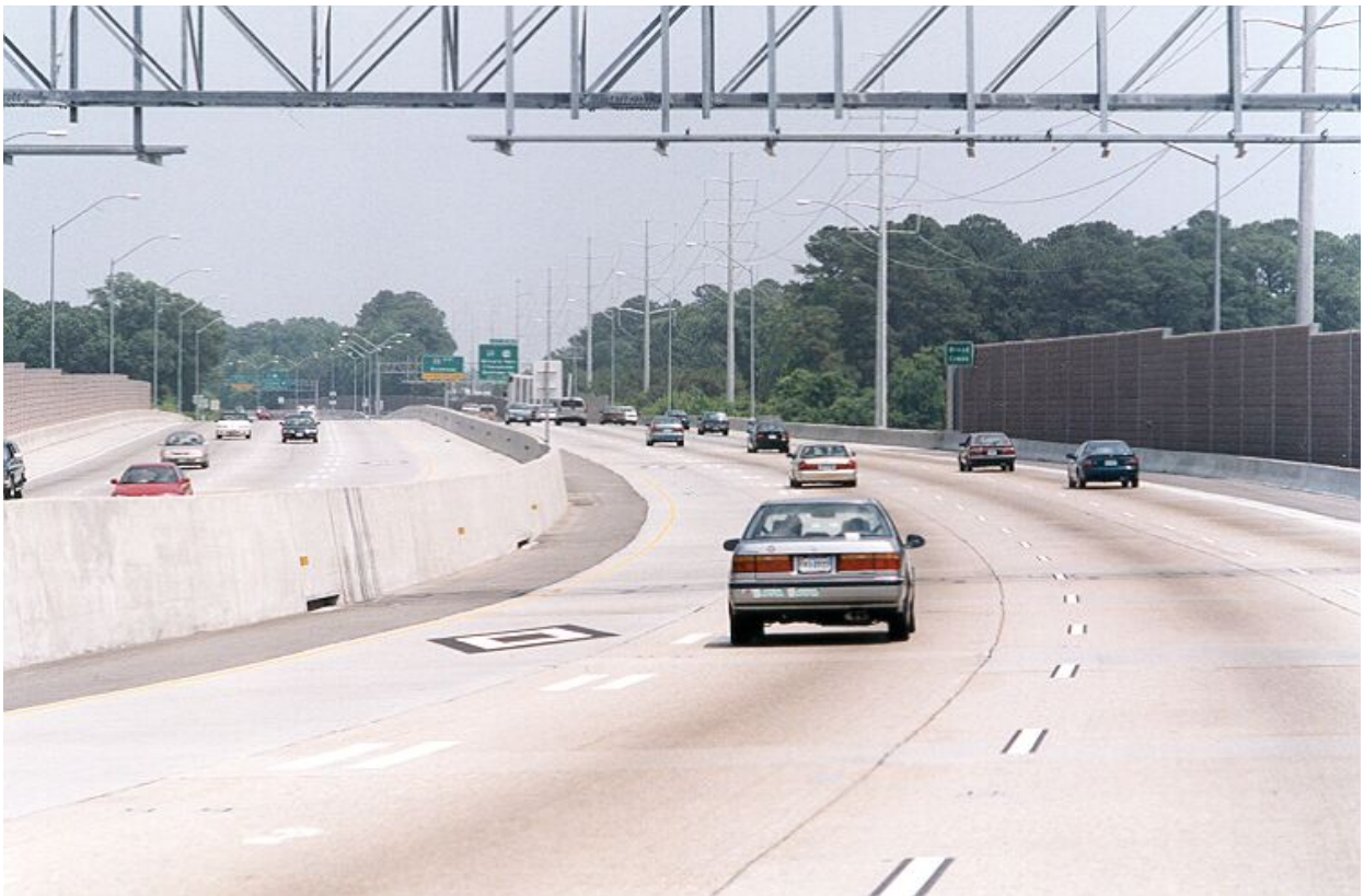
Figure 1. Concrete median barrier on a narrow median suburban highway with high traffic volume.
