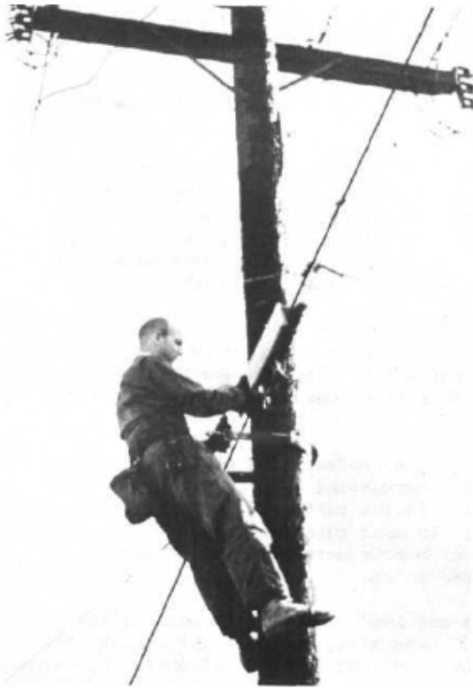
Figure 2. Diphacin bait blocks being attached to a utility pole above the telephone cable. The terminal is adjacent to the workers right arm.
