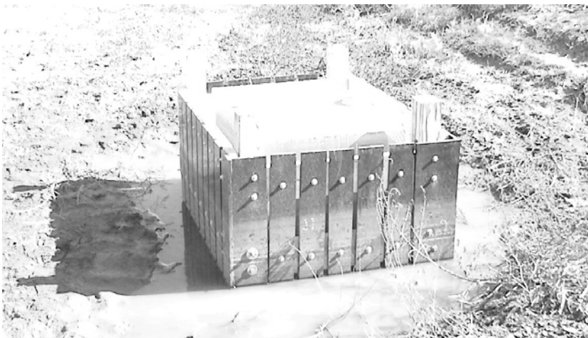
Figure 6. Inlet Strainer after Installation
