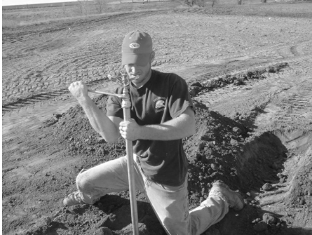
Figure 4. Sprinkler Riser Installation
