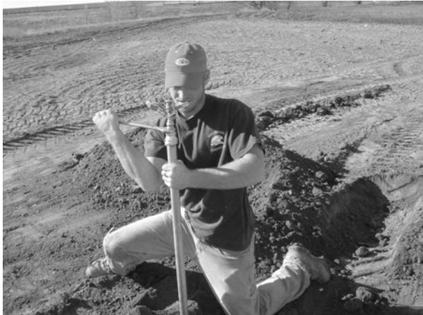
Figure 4. Sprinkler Riser Installation
