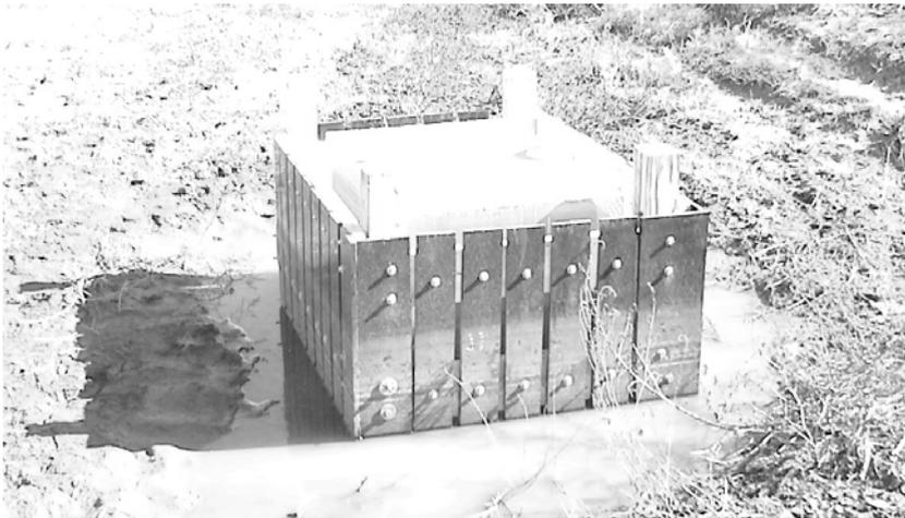
Figure 6. Inlet Strainer after Installation
