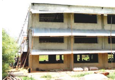
Multi-level poultry barn designed to improve air circulation near Maradi (upper) and poultry nutritionist Salissou Issa, INRAN visiting a poultry farm (lower) in Niger
