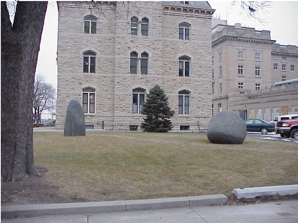
Image 10: Government Square Park Pre-2004 Renovation
