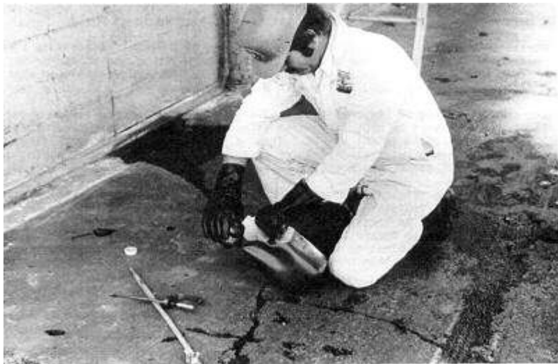
FIGURE 4. Filling trigger oil can with Rid-A-Bird solution. The service technician is wearing protective gloves as well as coveralls and hard hat.
