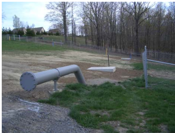
Figure 1. Access points for 12" Cased Pipe
