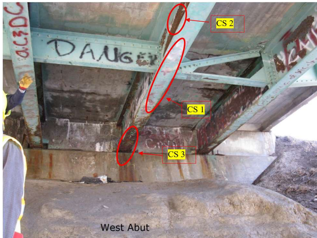
Figure 6.8 Bridge with multiple condition states
