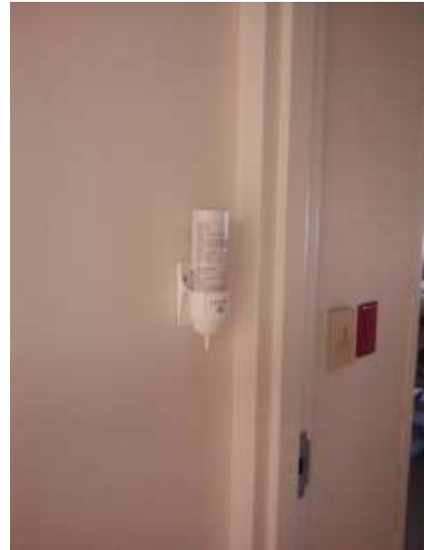
Figure 6-Antibacterial foam hand hygiene stations are added to the wall outside of the room.
