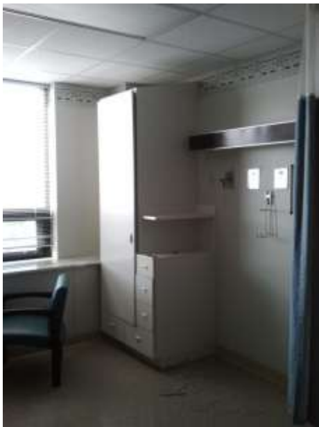
Figure 7-Shared patient room prior to remodeling.
