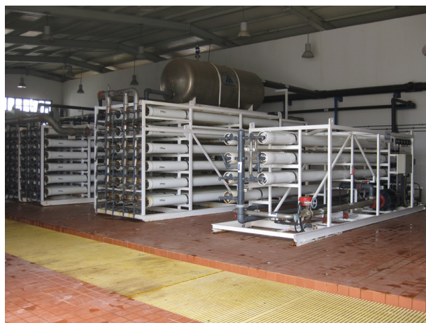
Figure 8. Dahab RO Membrane Unit
