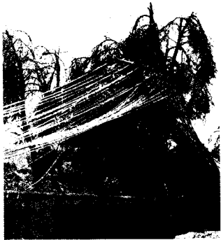
Sleet storm damages open wire telephone wires and poles. Poles were usually broken at ground level, with wires stretched and sagging; both poles and wire usually had to be replaced complete. (1915-1920)
