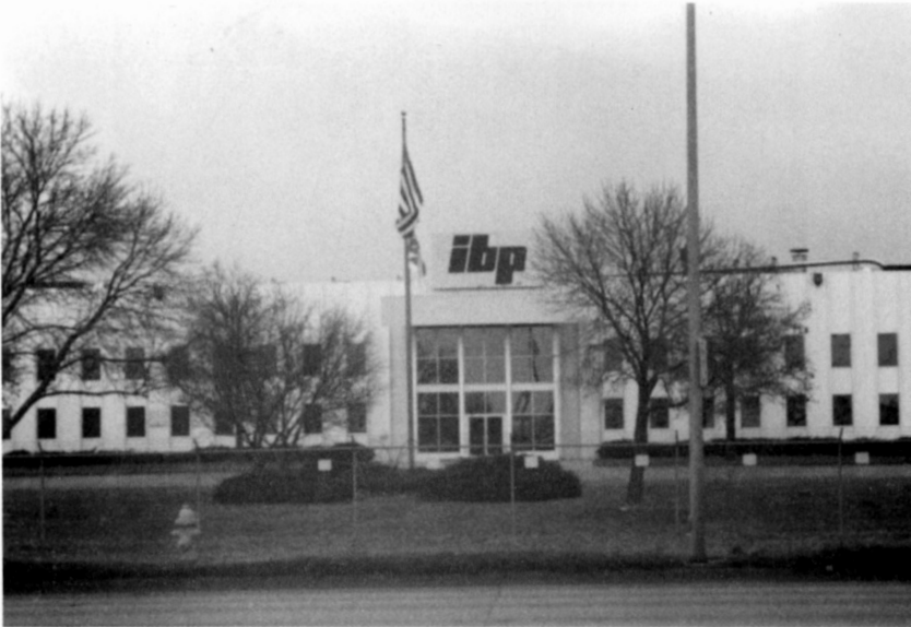
Figure 4. IBP, Inc. This modern plant is located across the Missouri River in Council Bluffs. It, too, hires many Latino newcomers. The plants are in competition for workers, as Omaha has a low unemployment rate (just under 2.0%). Meatplants have begun to offer more benefits for workers, but the work is non-union. These are not the high-paying union jobs of the old days. Also competing with the meatplants for workers are construction companies and telemarketing firms, the latter interested in those who are bilingual.
