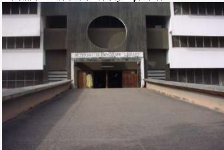
Fig. 1: Main entrance/front view of Hezekiah Oluwasanmi Library
