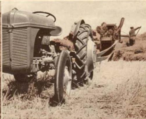
Smooth, even belt power for 22" x 36" separators, etc., without belt flap or overheating.
