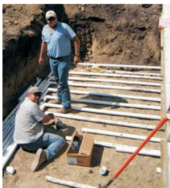
Connecting the main lines (beneath the control unit) to the manifold.
