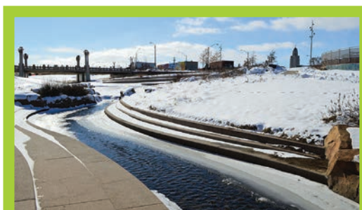
The City of Lincoln built a system to help manage Antelope Creek water flow and prevent flood damage through downtown Lincoln. The project was completed in 2012.
