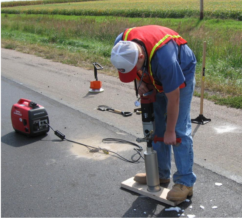
Figure 3.3: Use coring machine to drill cores
