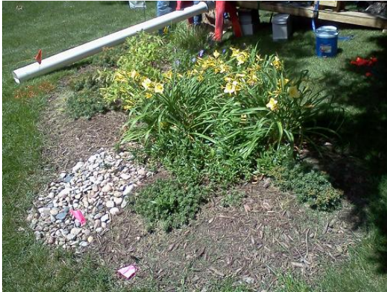
Figure 33. Rain garden installed on steep slope more than 30 ft. from downspout. Note heavily rock-armored overflow weir
