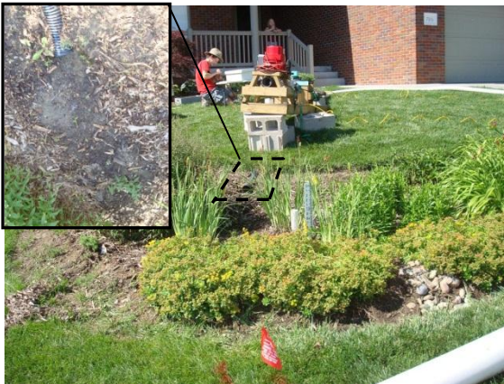
Figure 35. Rain garden connected to roof by buried black corrugated pipe emerging at the top slope of the cell. Insert photo shows closer look at inlet, which shows evidence of scour and sedimentation. Note the severe slope of the yard, which poses a challenge to residential rain garden performance.
