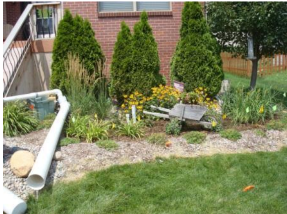
Figure 47. Inundated rain garden hugging foundation of home. Two roof downspouts contribute influent flow on either side of the garden.
