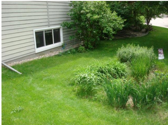
Figure 31. Densely vegetated rain garden with downspout shown as influent water source.
