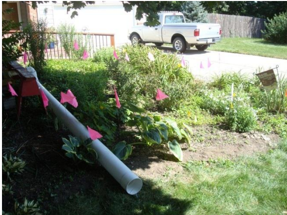
Figure 43. Previous rockbed and water feature converted to a rain garden. Poor berm definition and lack of berm near the driveway characterize this site.
