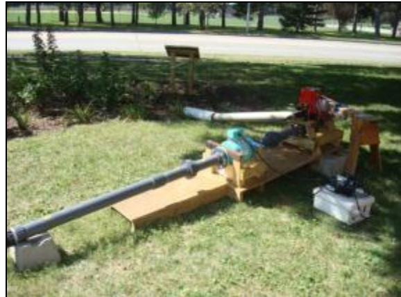
Flow meter/valve delivery system at inlet(9/23/10)
