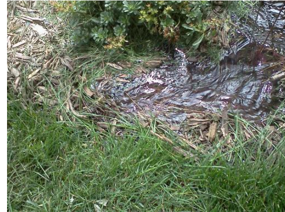
Figure 34. Improper outflow location observed, leading to mulch and soil erosion
