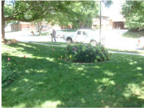
Figure 45. Rain garden at bottom of steep yard slope, not connected to downspout flow. Note large amounts of shade present.
