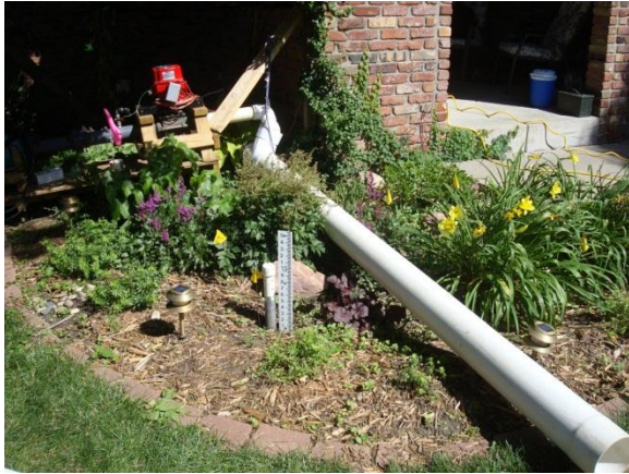
Figure 37. Rain garden close to the foundation which receives influent from vine-covered downspout on brick wall. White pipe directs water leaking from valve out of garden before test is conducted.
