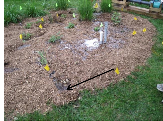
Figure 30. Full rain garden characterized by floating mulch. Overflow can be seen in foreground (see arrow),
