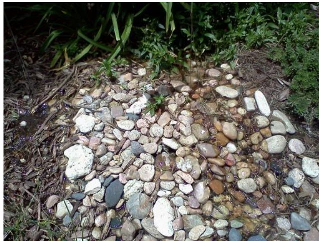
Figure 23. Photograph of proper site 5 rain garden weir overflow during simulated overflow storm (event 2). Note wet sheen on rock weir where water is flowing.
