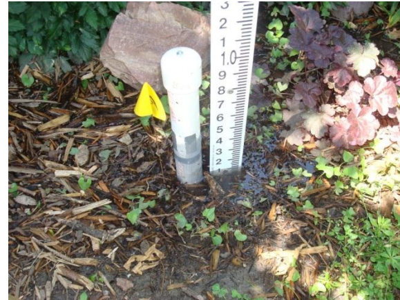
Figure 38. Stilling well containing transducer as well as staff gage. Slightly more than 0.1 ft. of ponding is occurring
