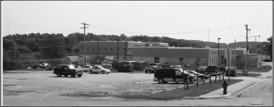
Figure 5-36. St. Clair County Jail. Photo by author.
