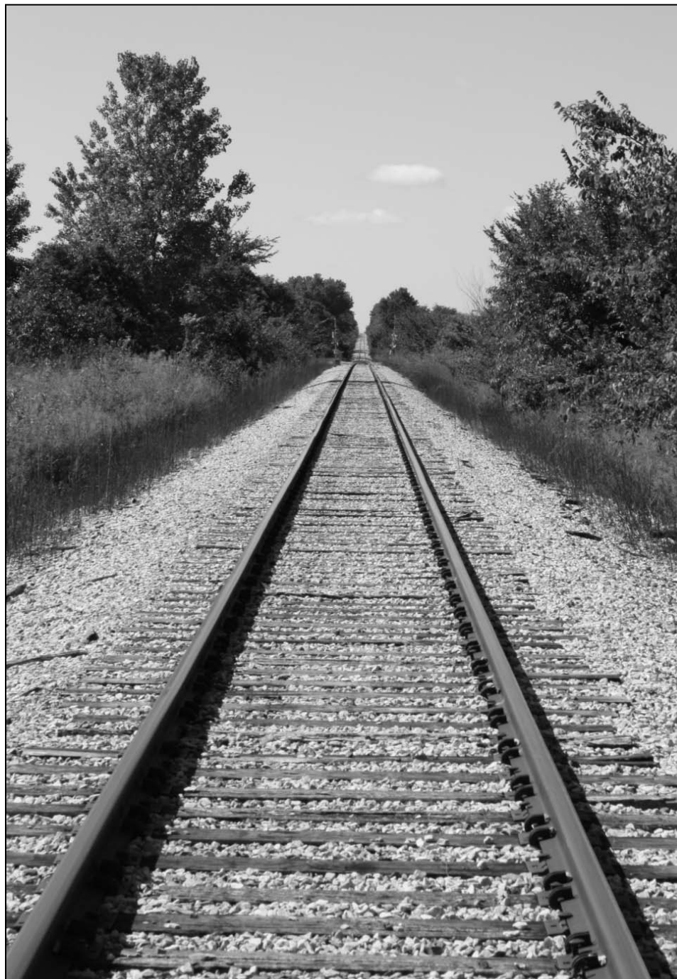
Figure 5-6. Abandoned MKT line south of Appleton City. Photo by author.
