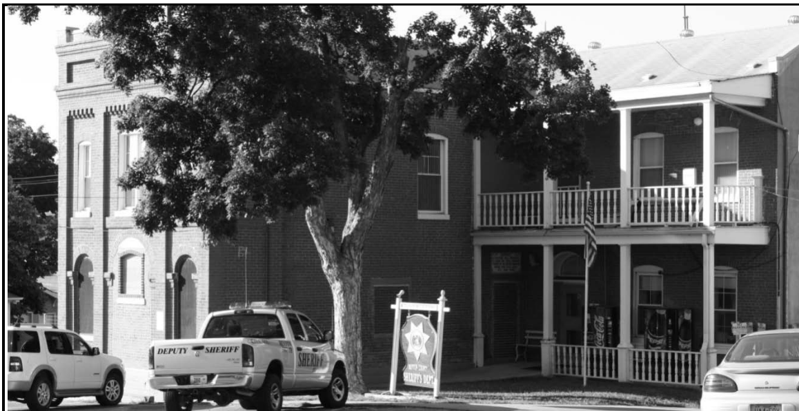
Figure 3-63. Benton County Jail. Another historic building serving a different purpose. Originally a bank building, built in 1856, the structure has served as the jail since 1912. Photo by author.
