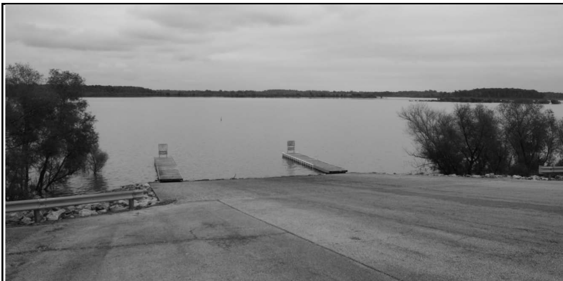
Figure 4-49. Boat launching ramp in Sparrowfoot Park. The Truman lake at the time of the photo is approximately thirteen feet above normal pool. Photo by author.
