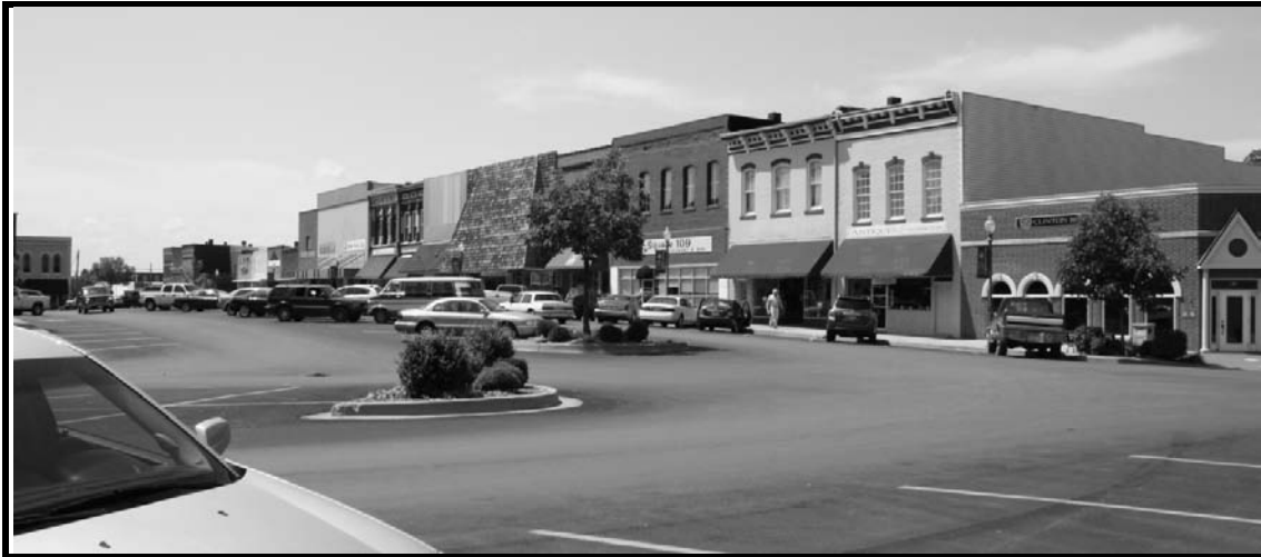
Figure 4-32. View of mostly retail businesses along the west side of Court House Square, Clinton. Photo by author.
