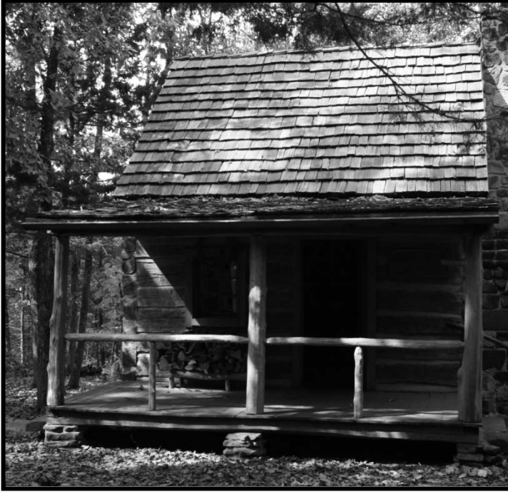
Figure 2-11. Ed Elmore Log Cabin at the Truman Visitor Center (constructed by volunteers associated with the Benton County Historical Society and Heritage Days volunteers.) Mr. Elmore was the first Truman project manager and later the first director of the visitor center. Photo by author.
