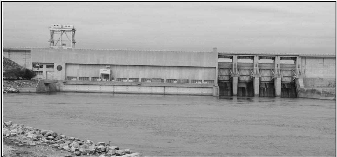
Figure 2-8. Truman powerhouse and spillway which is located on the left side of the dam looking upstream. Photo by author.
