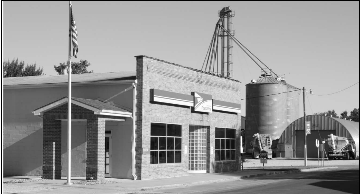
Figure 5-4. Post Office and MFA Elevator in Lowry City. Photo by author.
