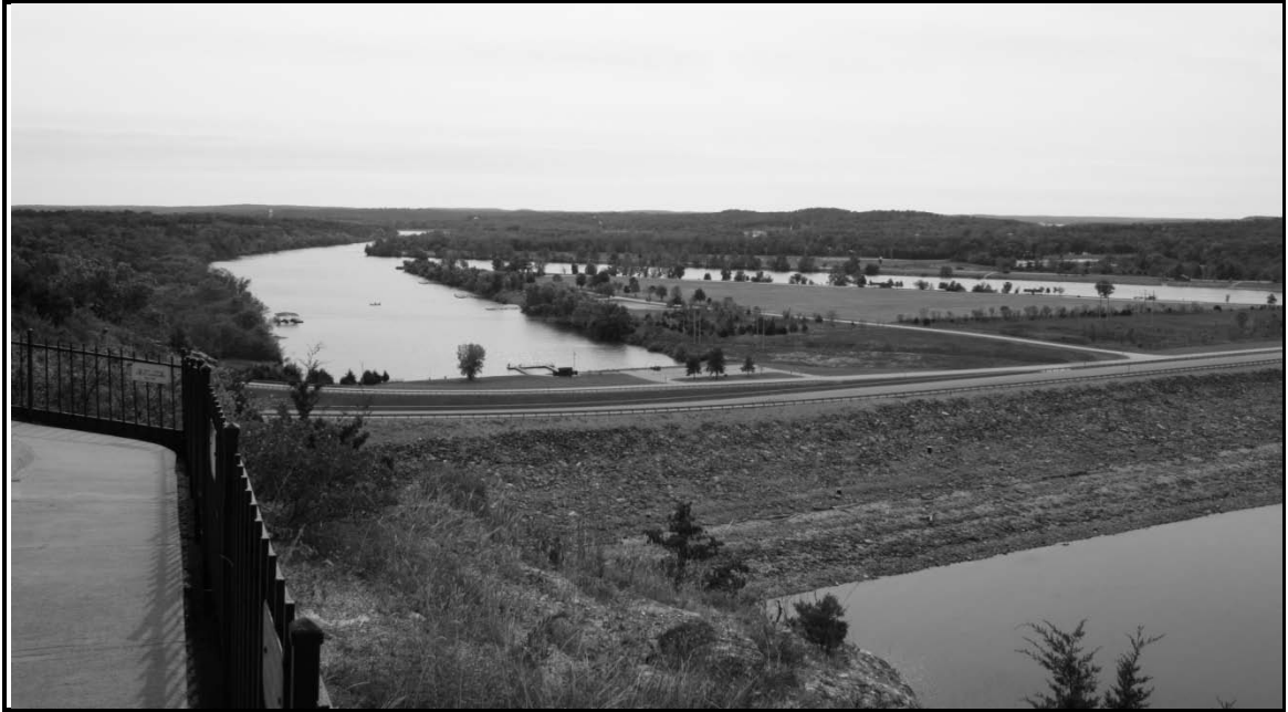
Figure 3-47. Approximately the same area viewed as Figure 3-46, but now from the Truman visitor center. Outlet channel for the power plant is to the far right the area just downstream of the dam is the remnant of Osage River (Lake of the Ozarks). Photo by author.
