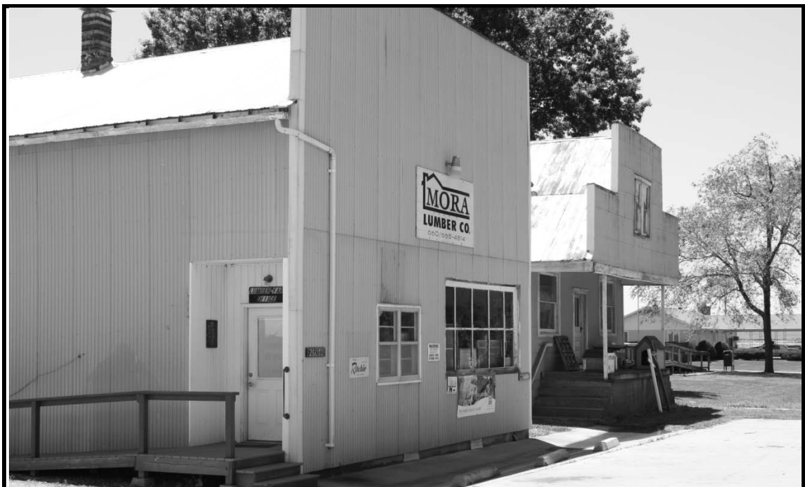
Figure 3-31. The lumber yard in Mora, located in northeastern Benton County. Photo by author.
