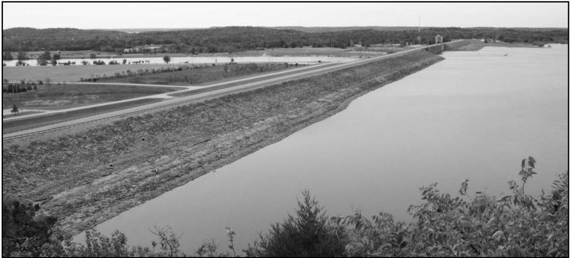
Figure 2-7. View of the Truman dam from the upper deck of the visitor Center. Powerhouse is located at the far end of the dam, outlet channel is located in the upper right. Photo by author.
