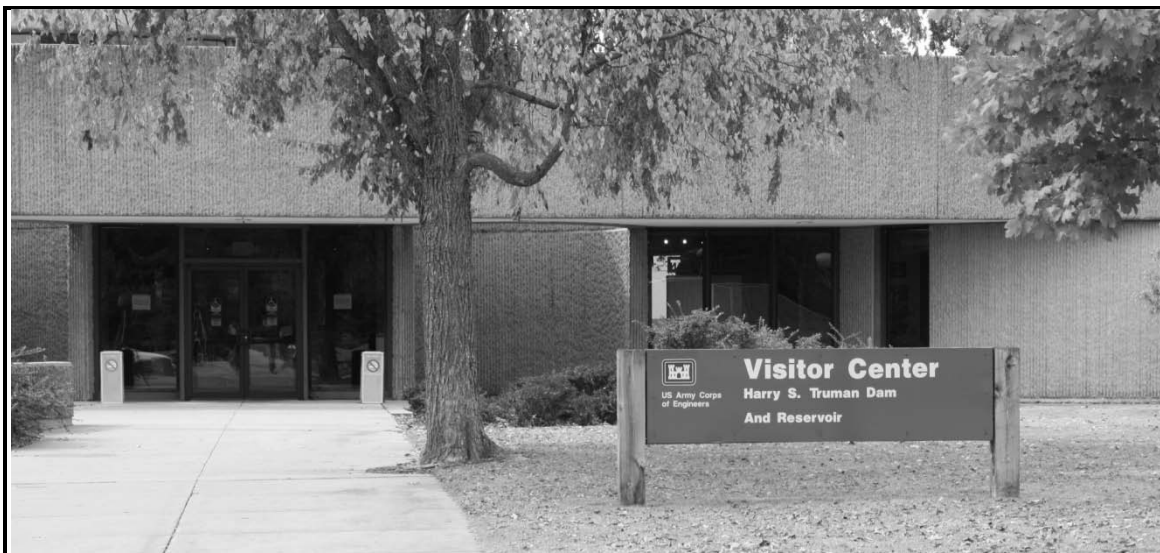
Figure 3-51. Entrance to the visitor center at Kaysinger Bluff Park. The center not only offers interpretive displays but a panoramic view of the project from Kaysinger Bluff. Photo by author.
