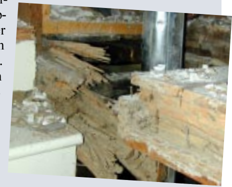
Termite swarms (above) in a Lincoln home with an extensive termite infestation. There was more than $30,000 of damage to the house, including a destroyed house beam (below).
