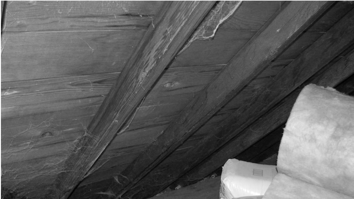
Figure 14 – BPI inspection of interior conditions
