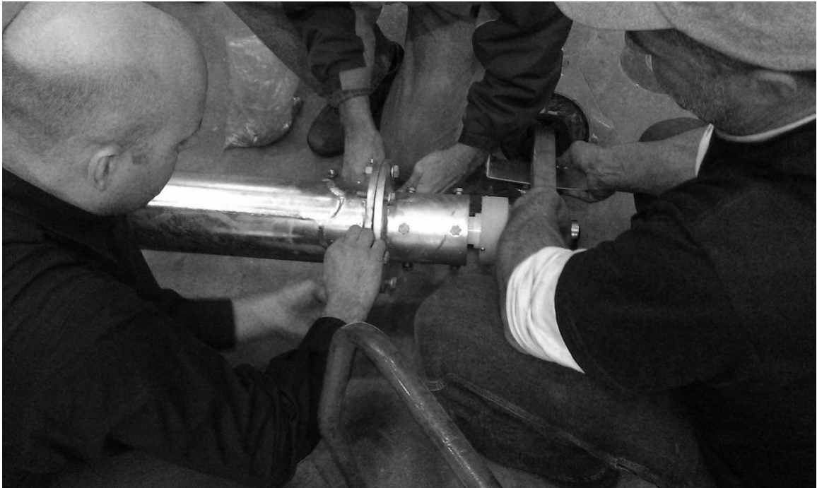
Figure 17 – Assembly of wind turbine
