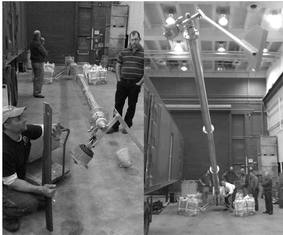
Figure 18 – Temporary erection of wind turbine
