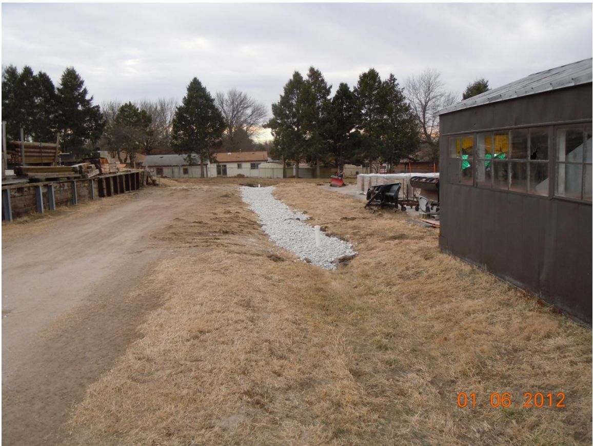
Figure B.5 Infiltration trench after construction
