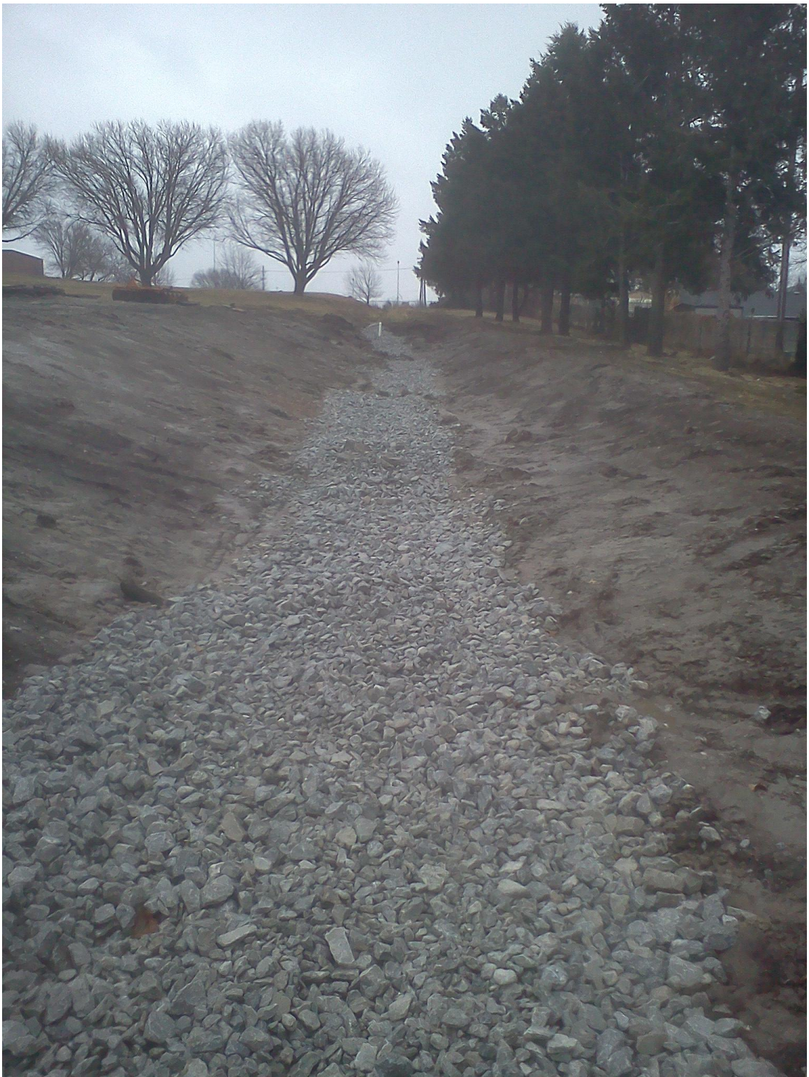
Figure B.7 Filter trench after construction
