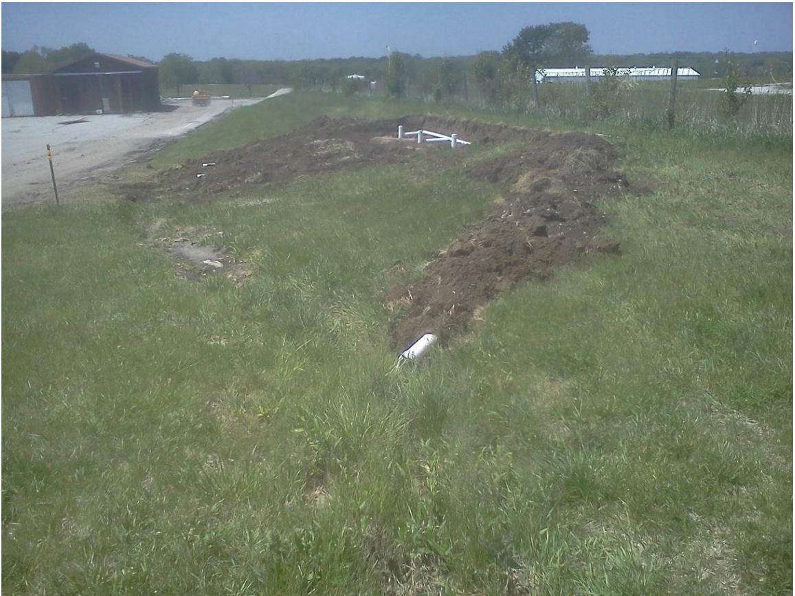
Figure B.8 Bioretention diversion during construction
