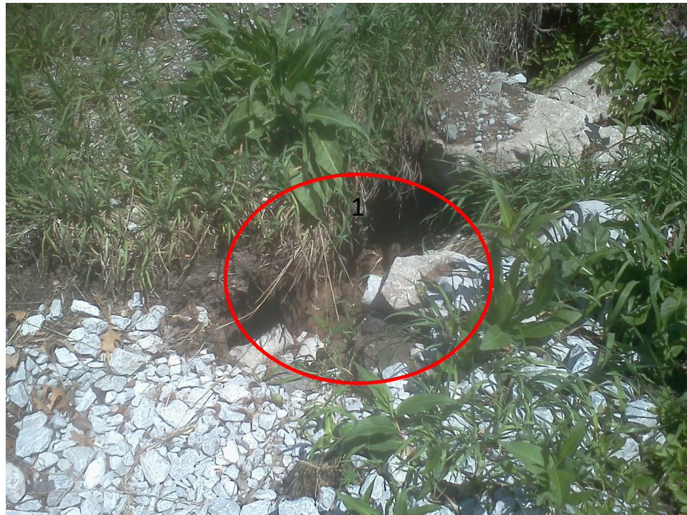
Figure 2.23 Filter trench undermining at beginning of trench
