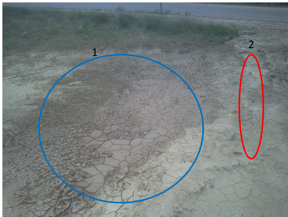
Figure 2.17 Check dam filter clogging
