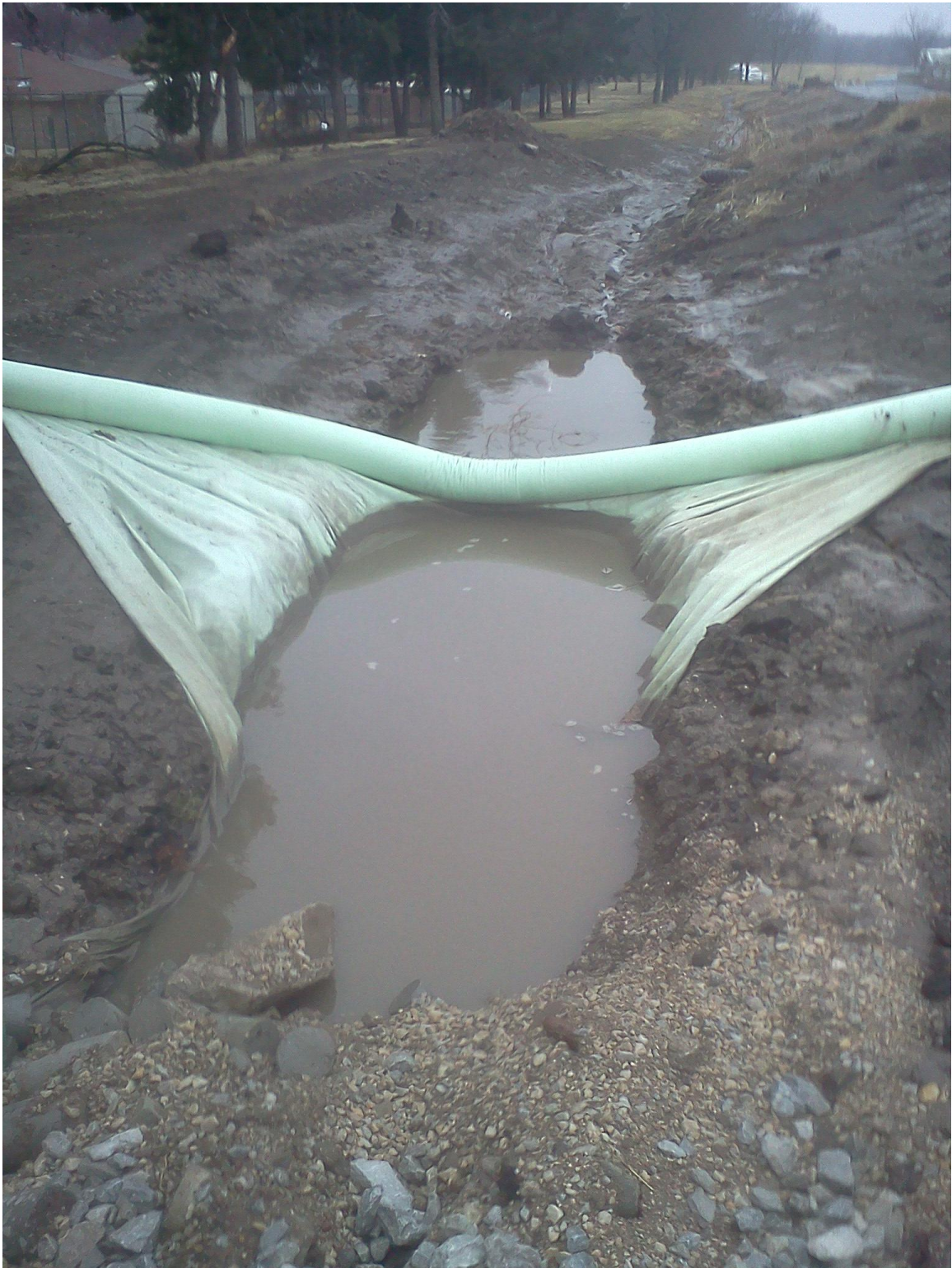
Figure B.11 Rain event during construction of filter trench
