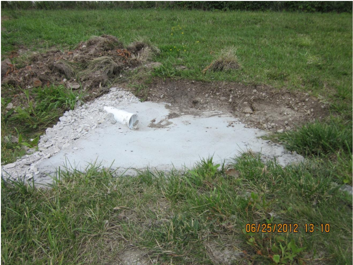
Figure B.9 Bioretention diversion after construction
