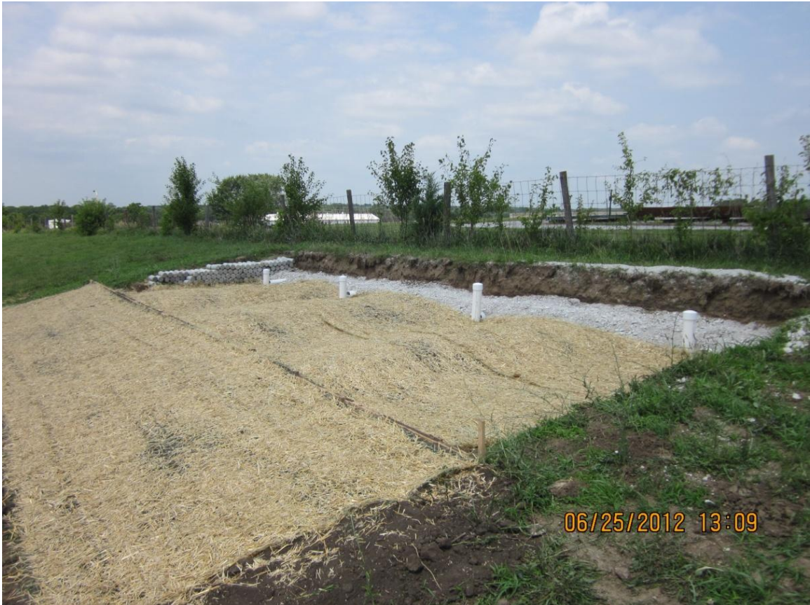
Figure B.1 Bioretention after construction
