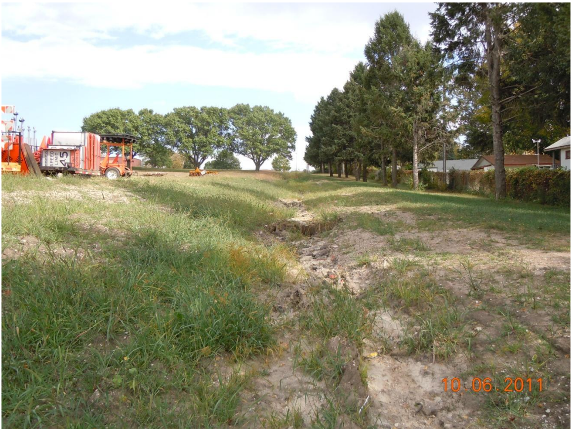
Figure B.6 Filter trench before construction
