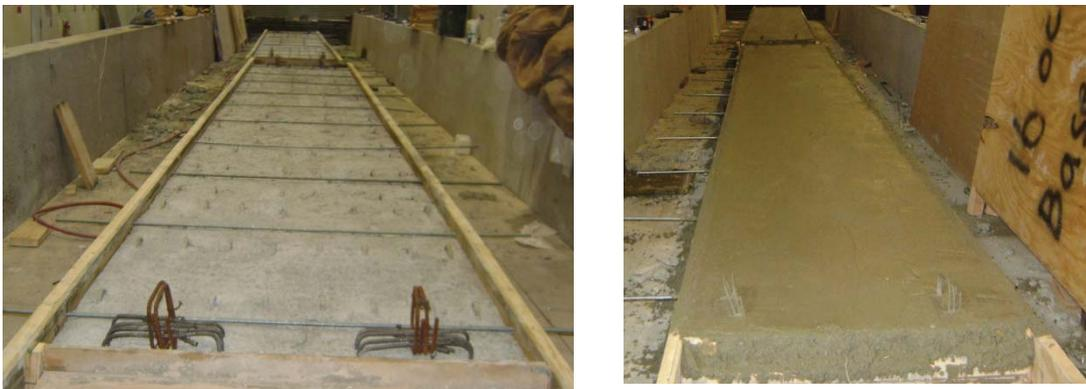
Figure 7.16: Built the form for the topping and cast the concrete topping
