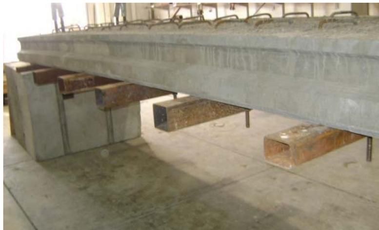
Placing the beam steel ledge and the temporary ledges
