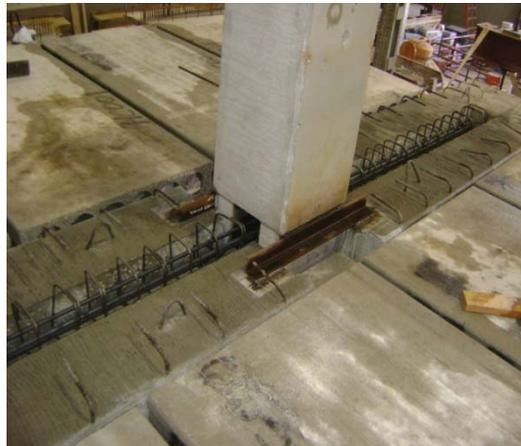
**Placing HC planks and pocket reinforcement**
