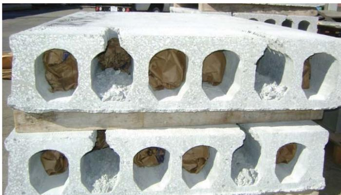
Figure 6.26: Blocking the HC openings before erection
