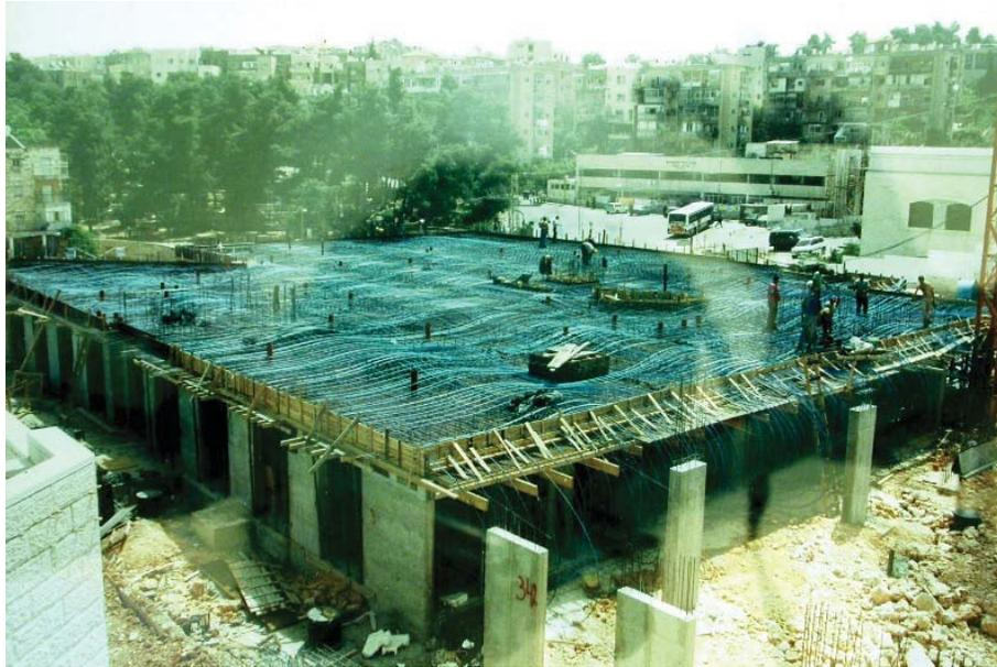
Figure 2.1: Construction of post-tensioned cast-in-place concrete slab
