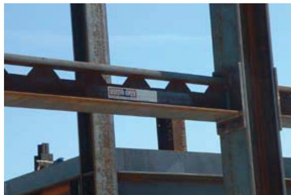
Figure 2.18: D-BEAM™, by Girder-Slab Technologies LLC, Cherry Hill, NJ (2002).
