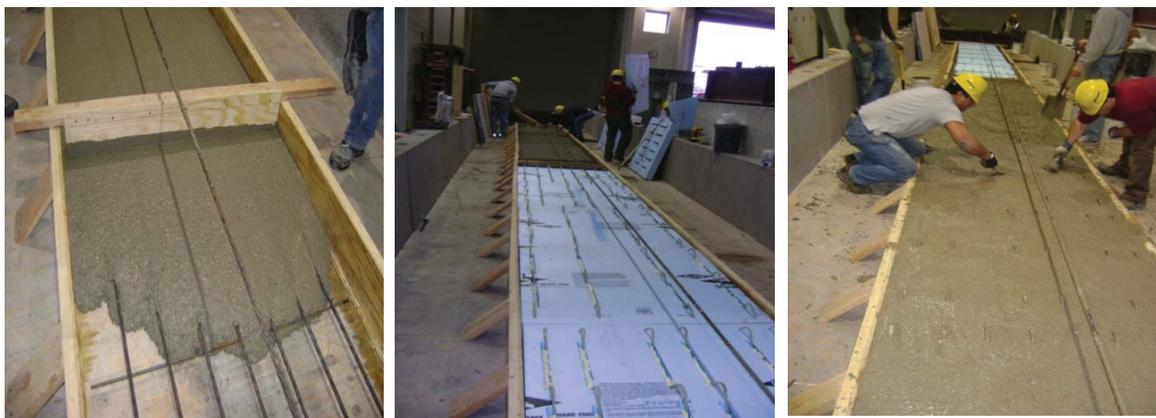
Figure 7.10: Casting the bottom wythe, installing foam panels, and casting the top wythe
