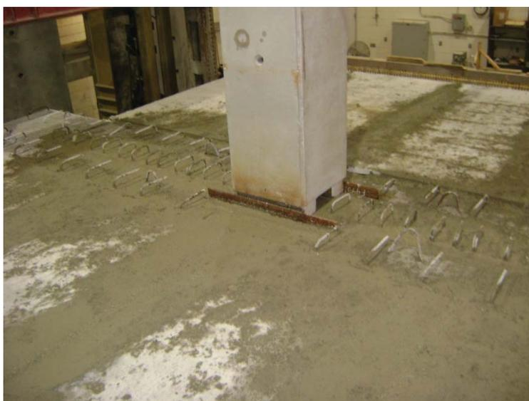
**Grouting the H.C keys and beam pocket with SCC**
