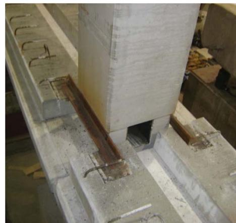
Welding the top angles to beam and column
