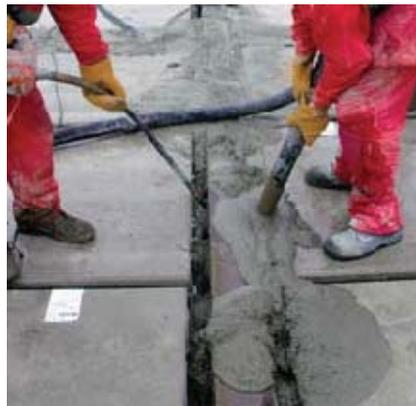
Figure 2.20: Filling the Deltabeam with self-consolidating concrete.
