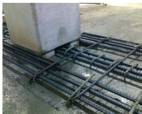
**Placing the topping reinforcement and C-bars**
