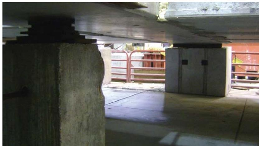
**Remove temporary corbels after the topping hardening**
