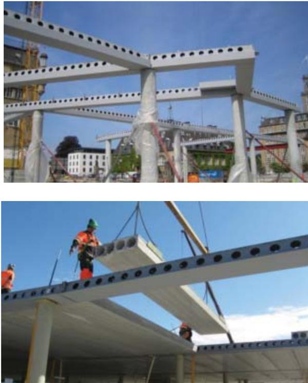
Figure 2.21: Construction of Deltabeam floor system.
