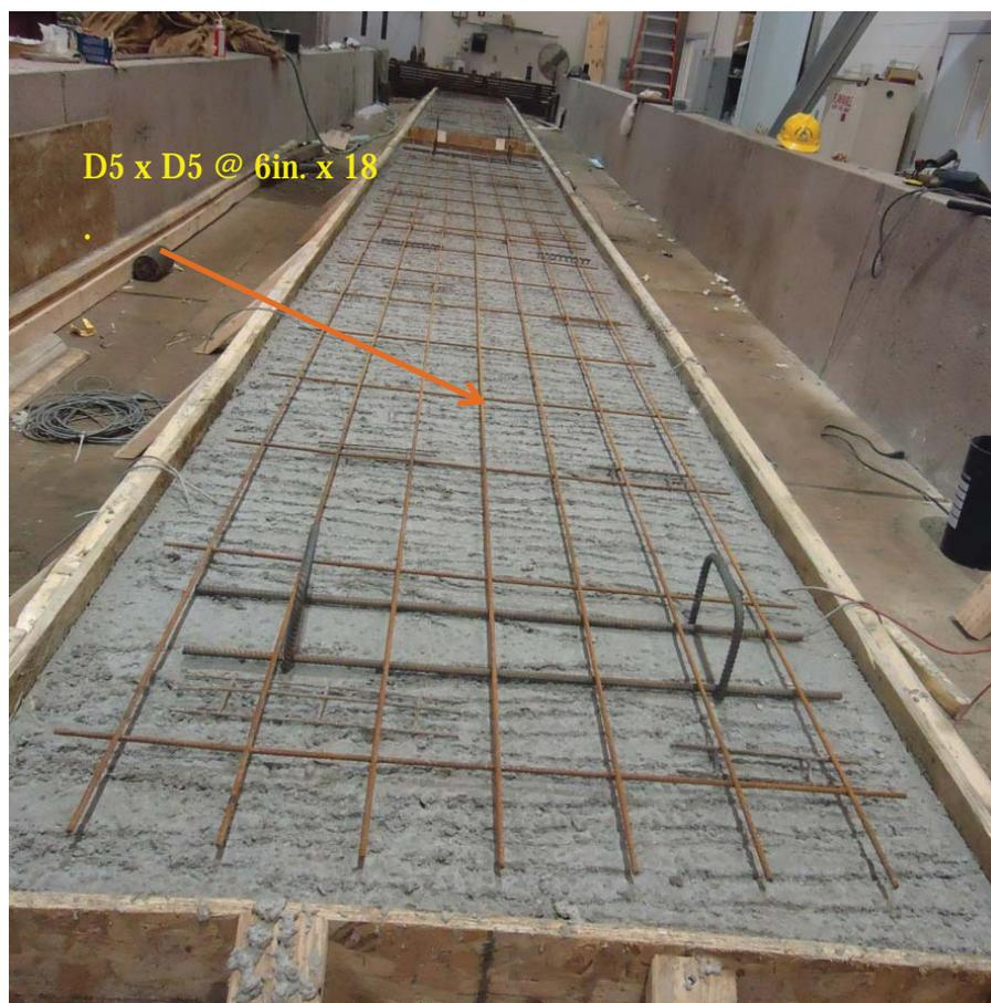
Figure 7.25: Topping reinforcement phase I (top) and phase II (bottom).
