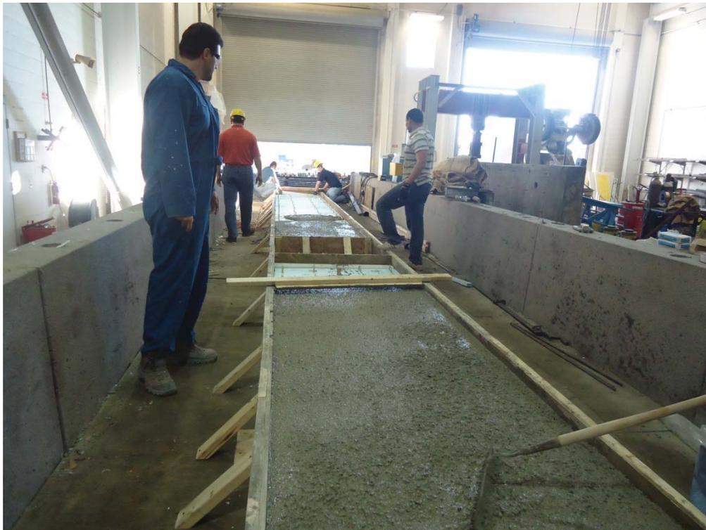
**Casting the bottom wythe, installing foam panels, and casting the top wythe**
