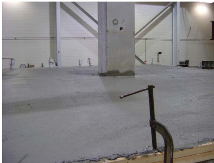
**Pouring and finishing the topping concrete**
