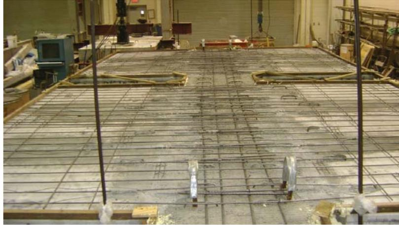
**Installation of welded wire reinforcement of the topping**
