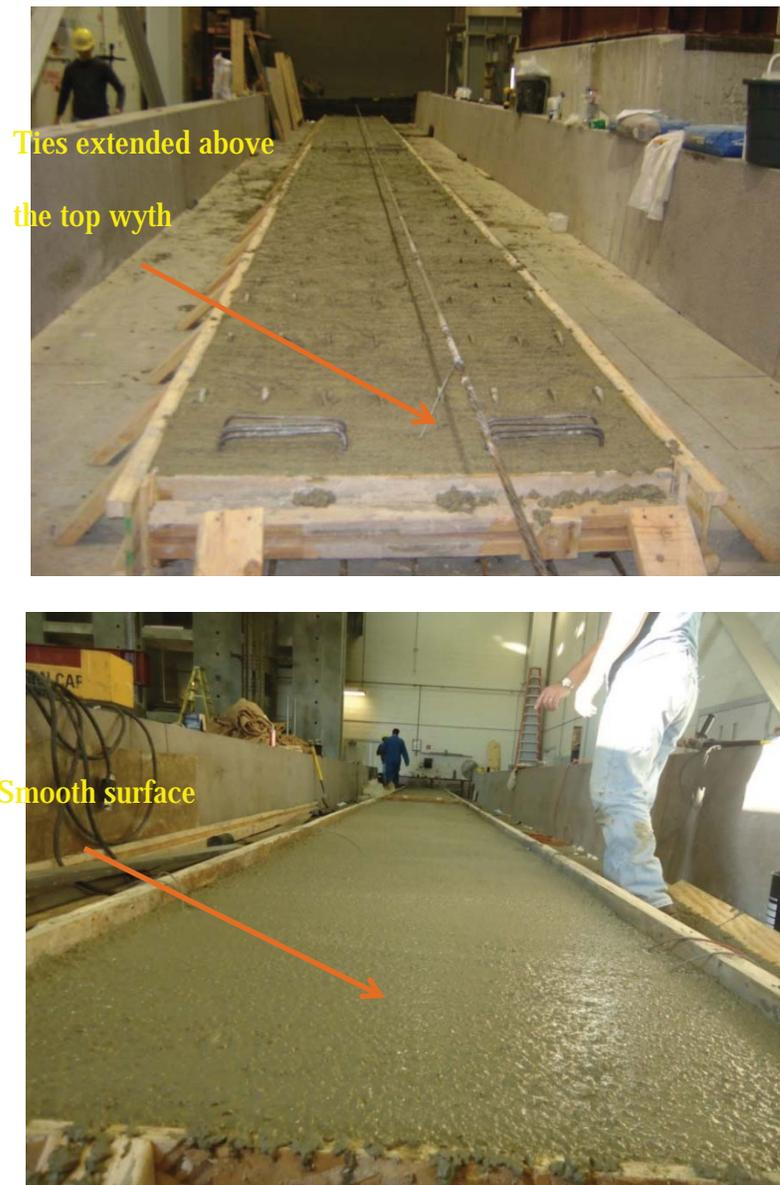
Figure 7.23: Changing the ties height in phase I (top) and phase II (bottom).
