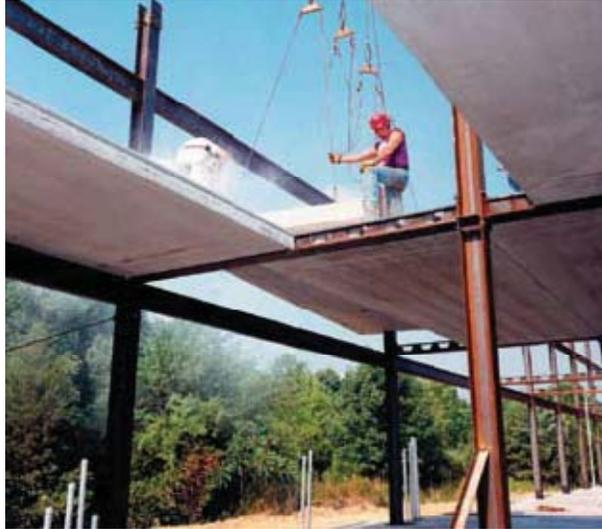
Figure 2.19: Construction using Girder-Slab system of Girder-Slab Technologies LLC
