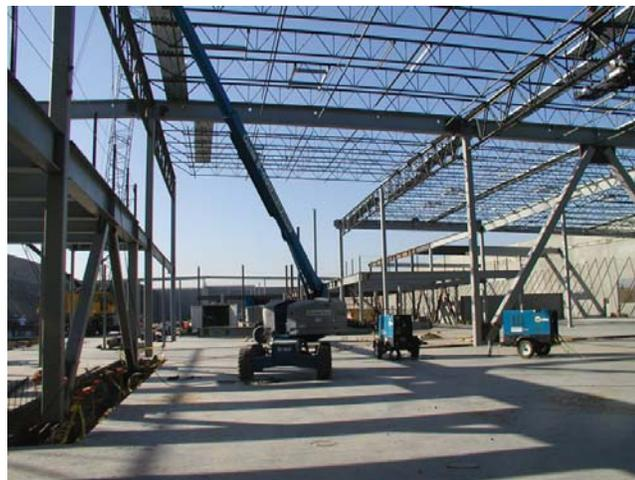
Figure 2.3: Construction of steel joist girder floor system
