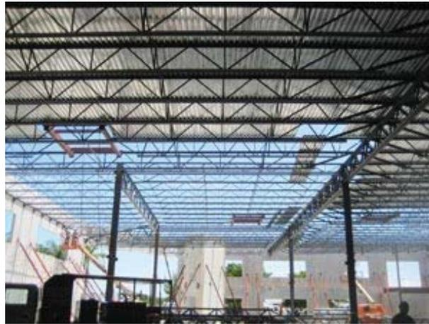
Figure 2.2: Construction of open-web steel joist floor system
