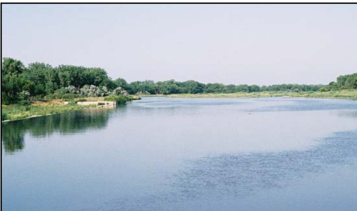
The Platte River at the Kearney Canal diversion dam.
