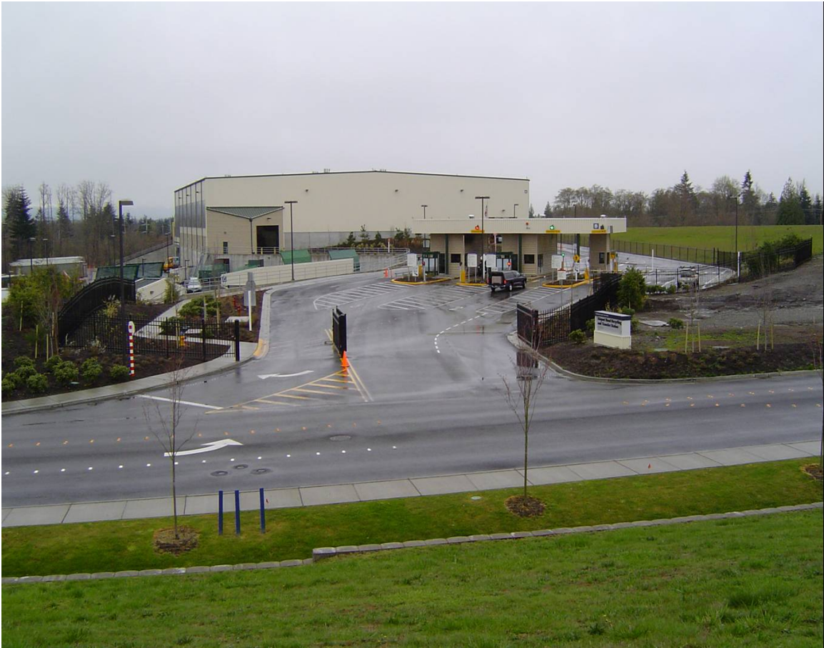
Figure 2. Photograph of the newly constructed and operational Airport Road Transfer Station at Paine Field, Washington.
