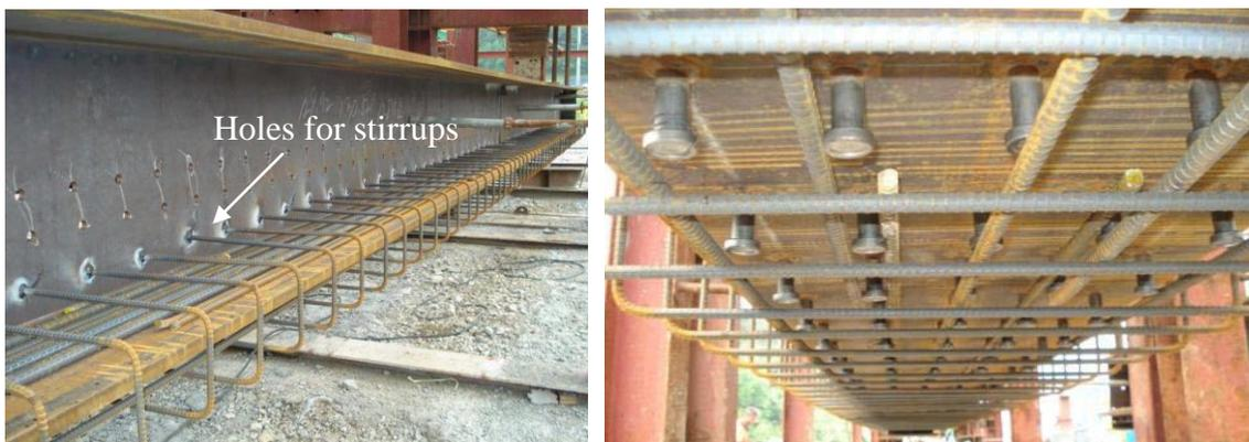
(b) Stirrups for Concrete Bottom Flange (Portela et al., 2011)
