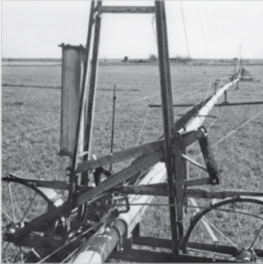
Figure 2.1. Original center pivot invented by Frank Zybach (Gaines, 2015)
