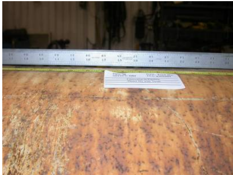
Figure 3-15. Defects D7, D8, D9 (p28dTH4)
