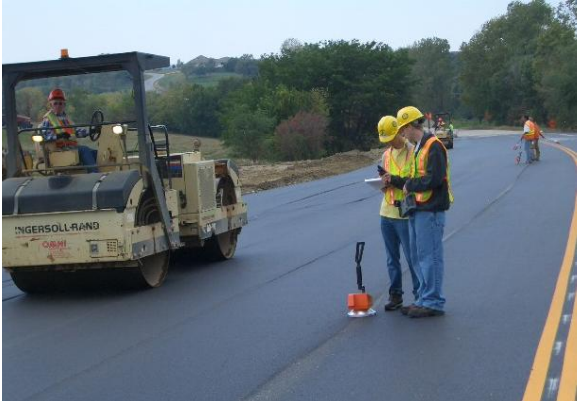
Figure 3.3 Taking PQI density readings onsite
