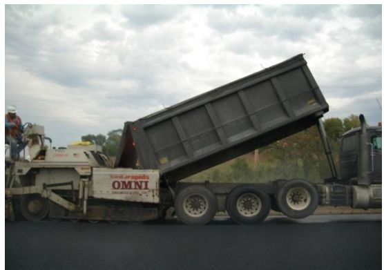
Figure 4.6 Direct dump between truck and paver
