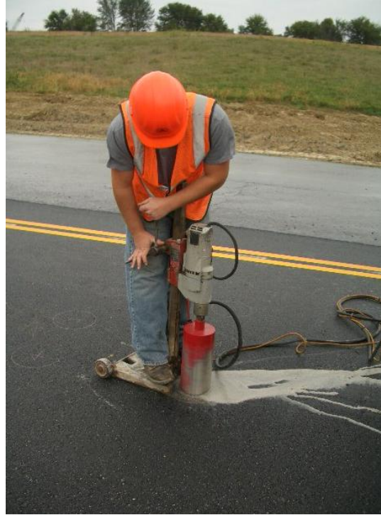
Figure 3.4 Taking cores for PQI calibration
