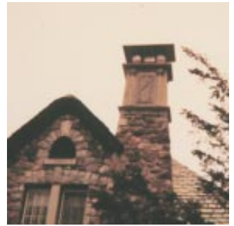
Chimney caps can prevent entry by summertime house guests.
