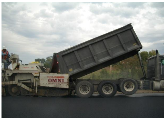
Figure 4.6 Direct Dump between Truck and Paver
