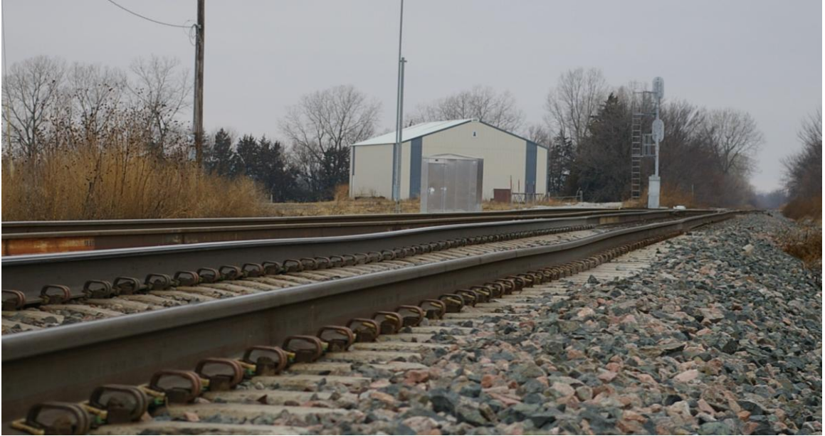
Figure 3-6. Geometry variation in track profile.
