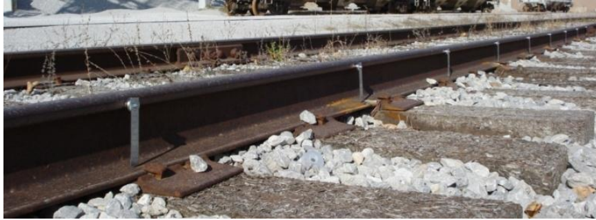
Figure 4-8. Magnetic rulers used to measure rail profile with surveyor's transit.
