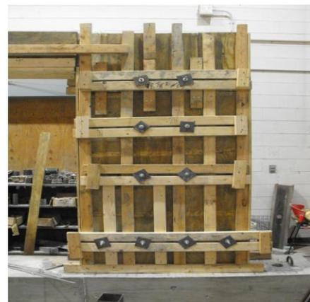
**Figure 3.33. Formwork Job Build Sustainable ICF Wall**
