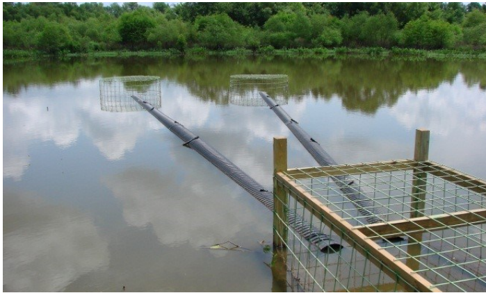
Figure 5. An example of a flow device using an exclusion fence at the culvert intake (lower right corner), corrugated pipes and round fences.
