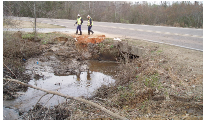
Figure 3. Beaver damage and the collapse of beaver dams can lead to structural damage of roadways and blocked culverts.
