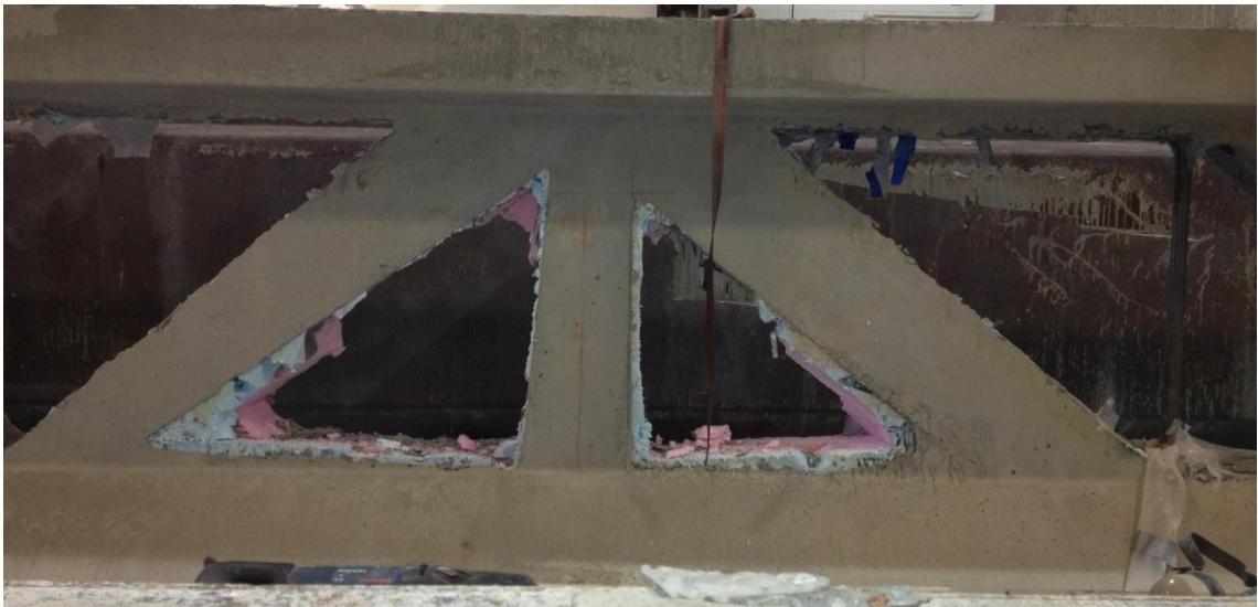
Figure 4.35 The middle of the truss after stripping the forms
