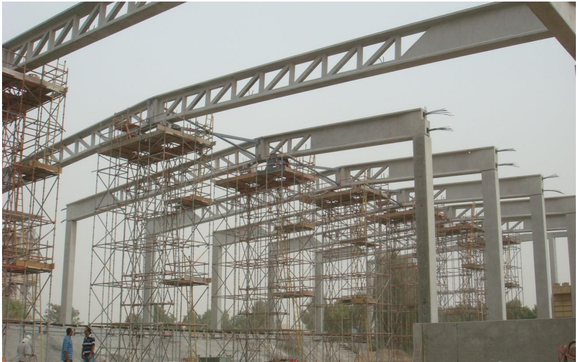
Figure 2.9 The trusses resting on the temporary supports before post-tensioning
