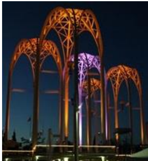
Figure 2.1 Concrete trusses Pavilion Science Center in Seattle, WA
