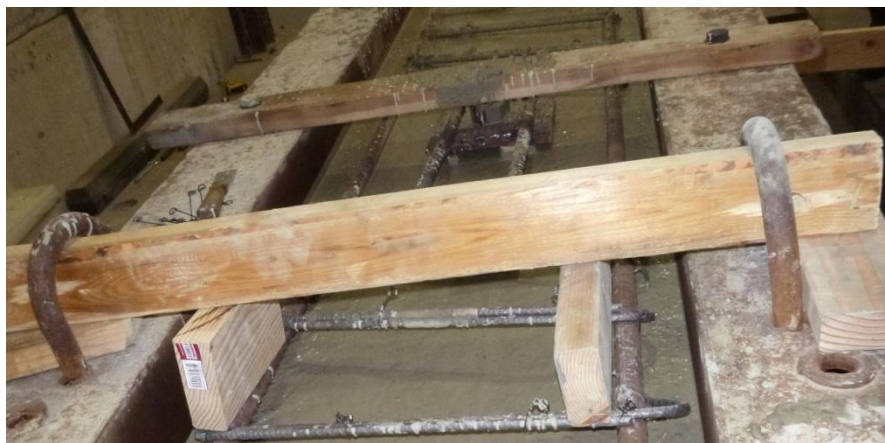
Figure 4.31 Holding down the steel reinforcements
