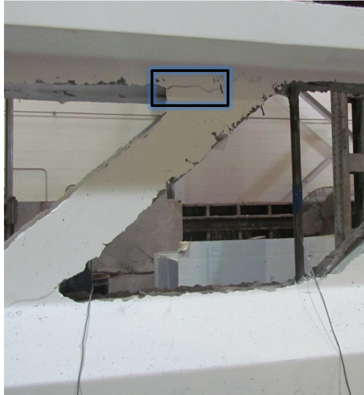
Figure 4.44 The only cracking that occurred at 100 kips of load.
