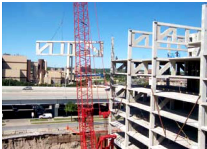
Figure 2.5 Erection of ER-POST trusses (Trygestad and DeSutter 2007)
