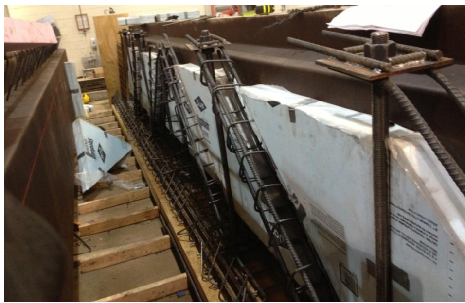
Figure 4.23 All the reinforcements after being fixed in the form
