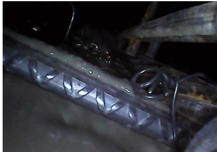
Figure 4.29 Snapshot from the south end recording while pouring
