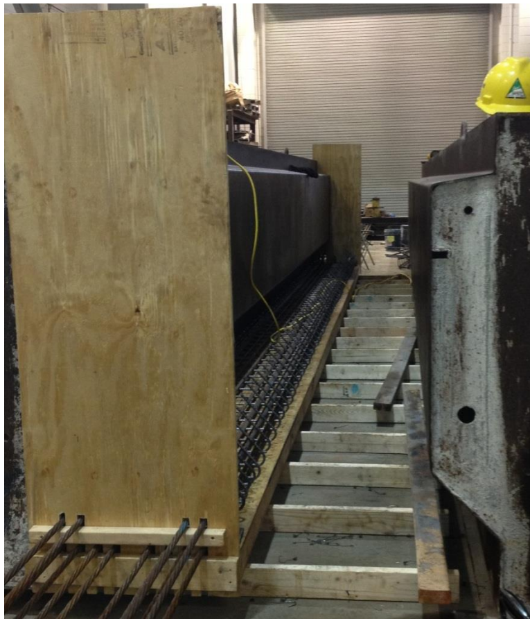
Figure 4.16 The strands after tying the stirrups and putting the end bulkheads
