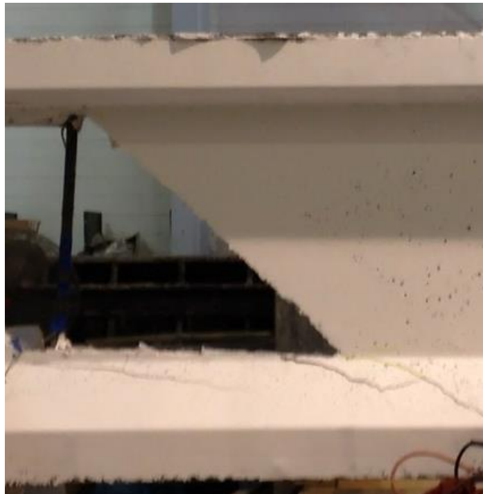
Figure 4.49 Excessive cracking right before and at location of failure
