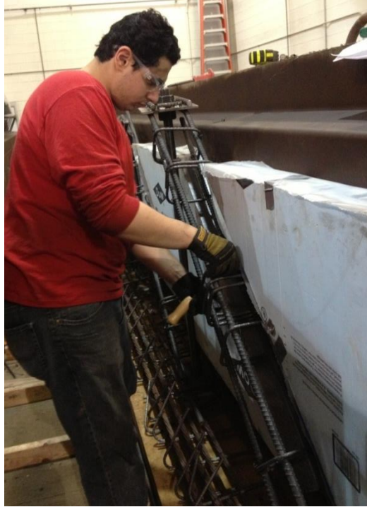
Figure 5.1 Tying the diagonal member reinforcements together after attaching the vertical
