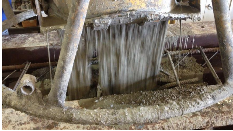
Figure 4.28 Pouring the concrete through the middle vertical member
