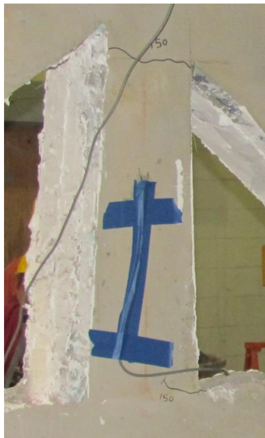
Figure 4.46 The middle vertical cracking at the 150 kip loading point
