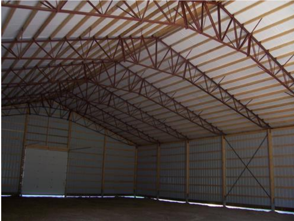
Figure 1.1 Interior of steel truss warehouse roof
