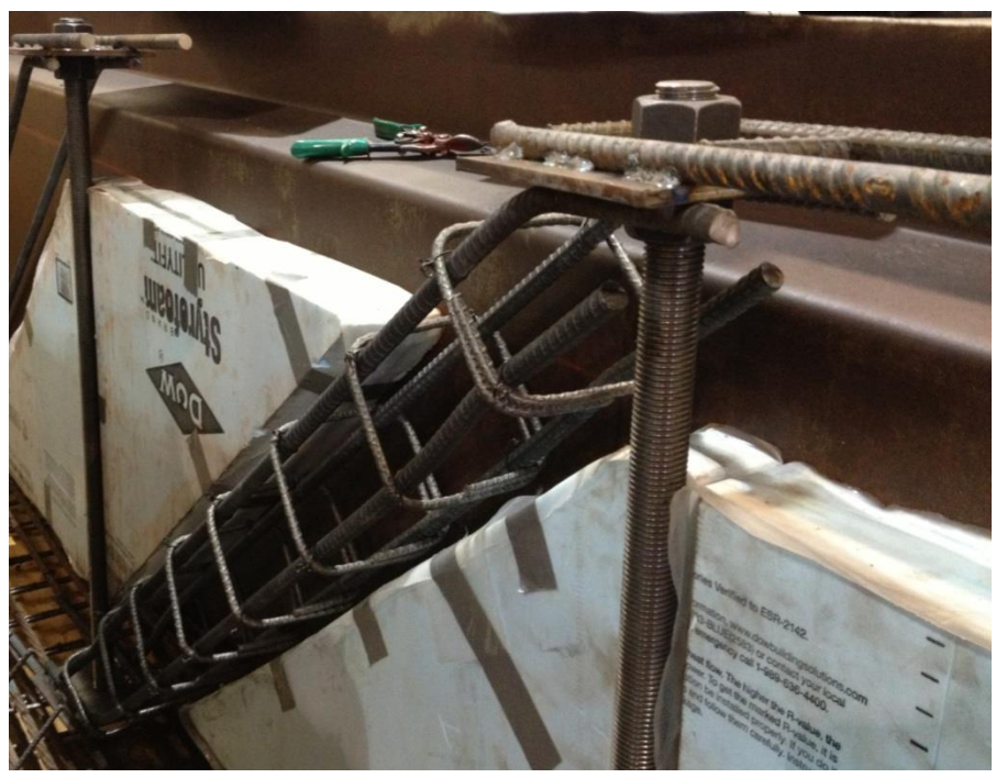
Figure 4.22 The diagonal reinforcement assembly
