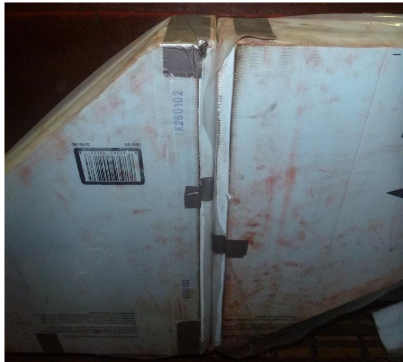
Figure 4.20 The groove and the plastics sheet on the block-outs
