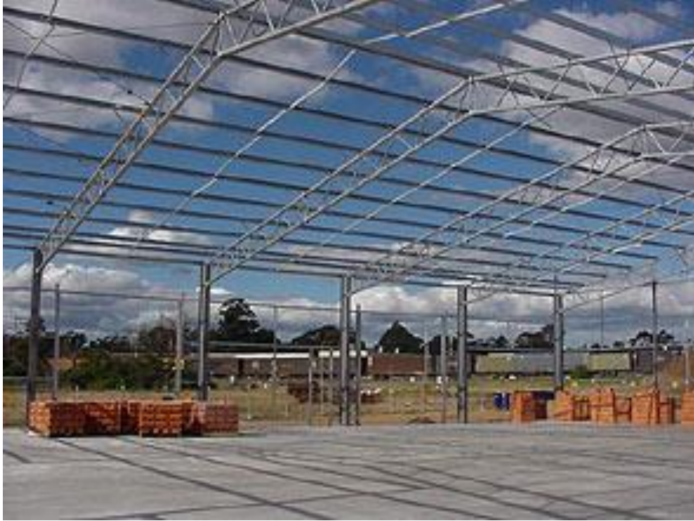
Figure 1.3 Steel trusses used for roof support
