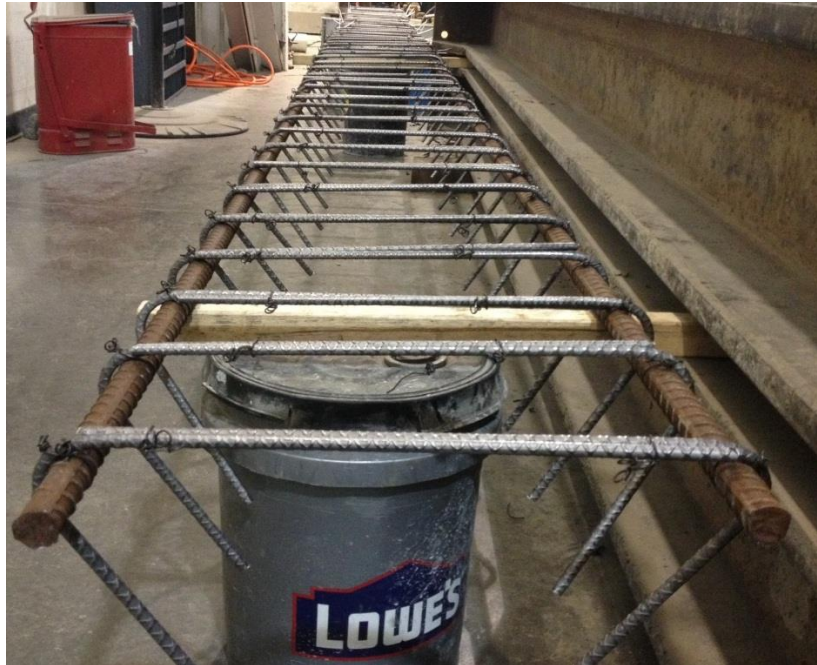
Figure 4.25 The top flange reinforcements after assembly
