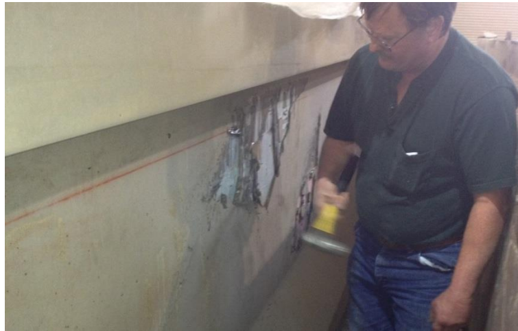
Figure 4.33 Chipping out the concrete layers covering the block-outs
