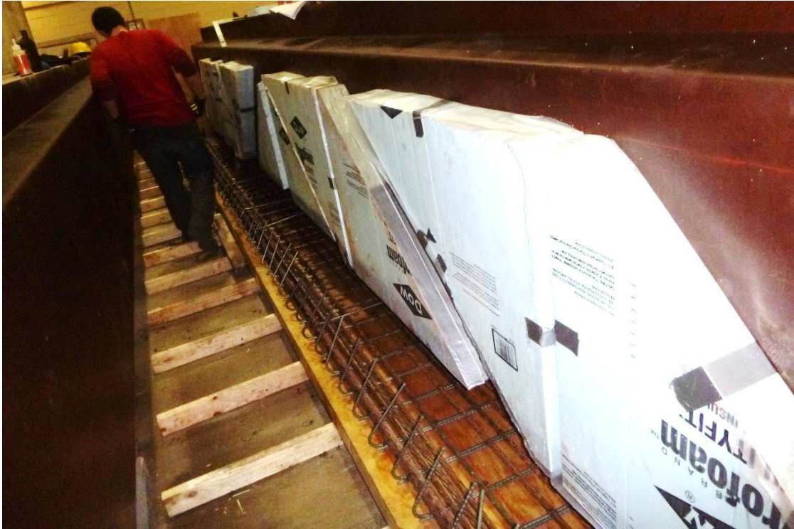
Figure 4.21 The Styrofoam block-outs after being glued on the steel form
