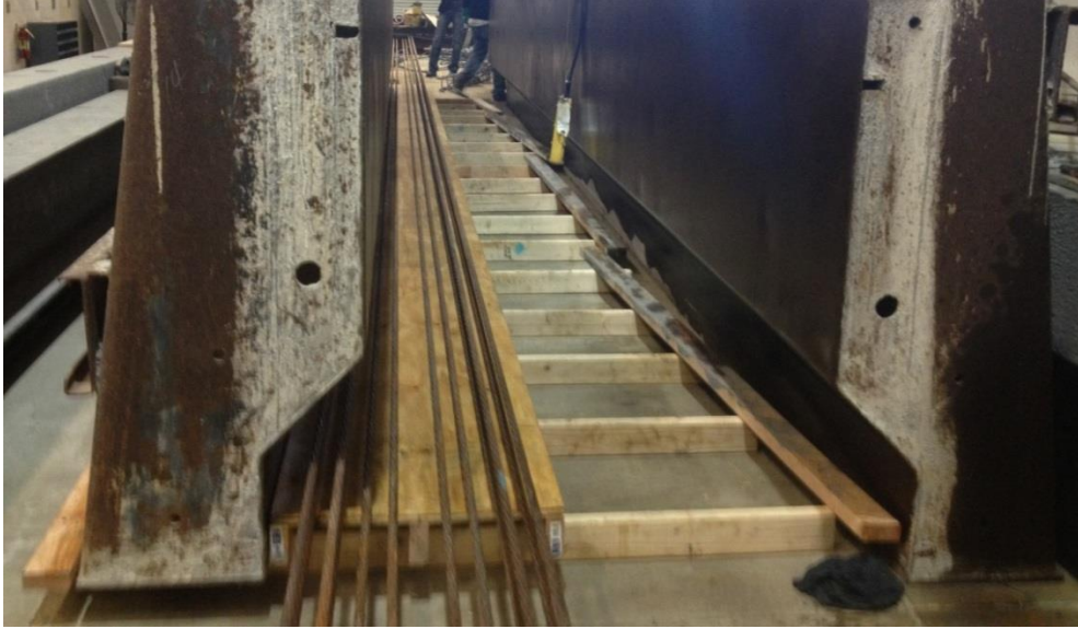
Figure 4.15 Fixing one side of the form in place
