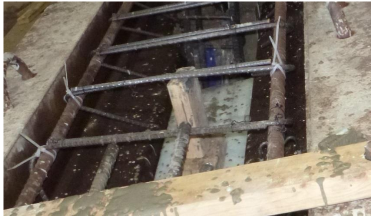
Figure 4.30 Holding down the block-outs
