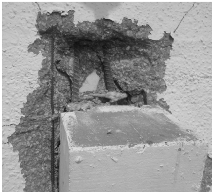
Figure 4-14: Ruptured NU-Ties in specimen A2
