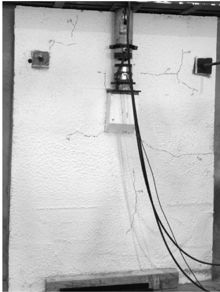
Figure 4-7: Marked plastic shrinkage cracks in specimen A1 prior to loading
