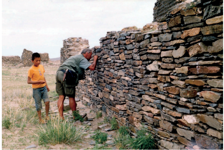
Fig. 2: K. Thiele exploring quarters of E. gobiensis and M. aurascens in wall cracks at Har Buhyn algas ruins. Photo: D. Dolch, 2002.
